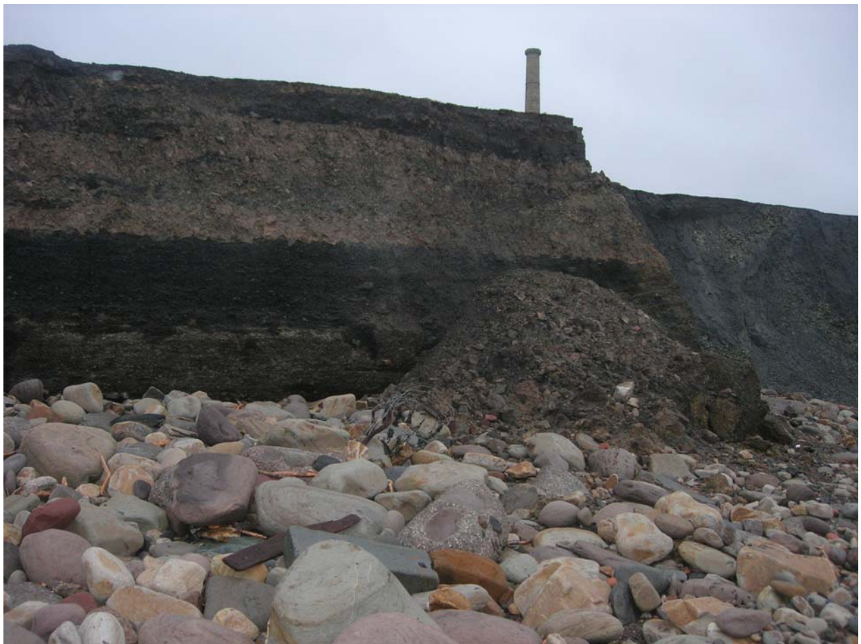
Figure 11. The fatal landslide (Landslide A) at NGR 296749 518380 (Photo: BGS, 03/01/07).
