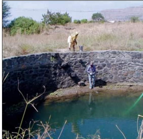
Photo A5.2 Large diameter well used for irrigation water supply, Kolwan Valley.
