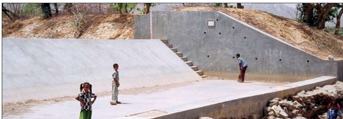
The downstream side of the Bhanavas check dam.
