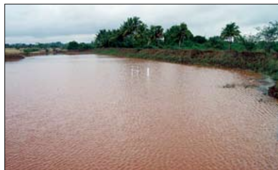
Photo A3.2 Automatic water level recording device in Karanampettai recharge structure when nearly full.
