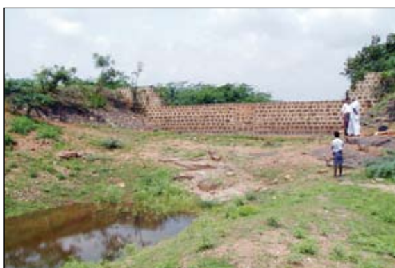
Photo A3.3 The Kodangipalayam West recharge structure received little water during the period monitored due to capture upstream.
