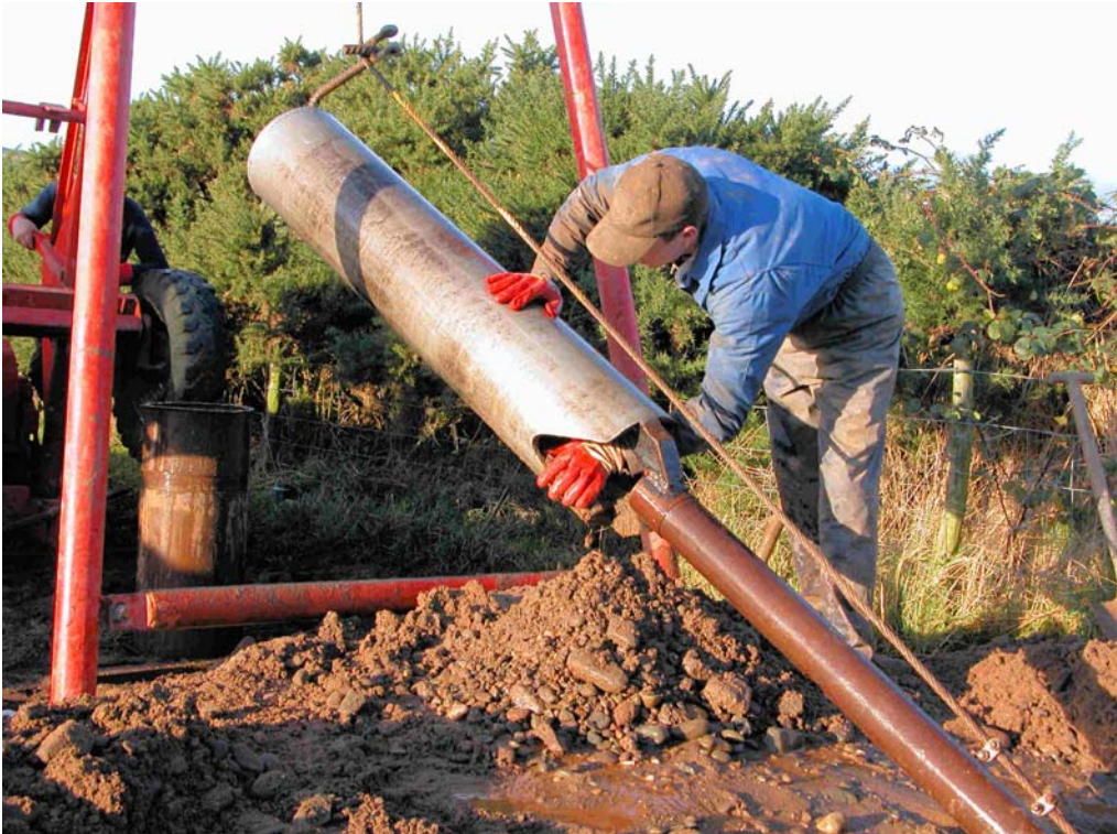
Figure 12 Emptying sand and gravel from the drill tool
