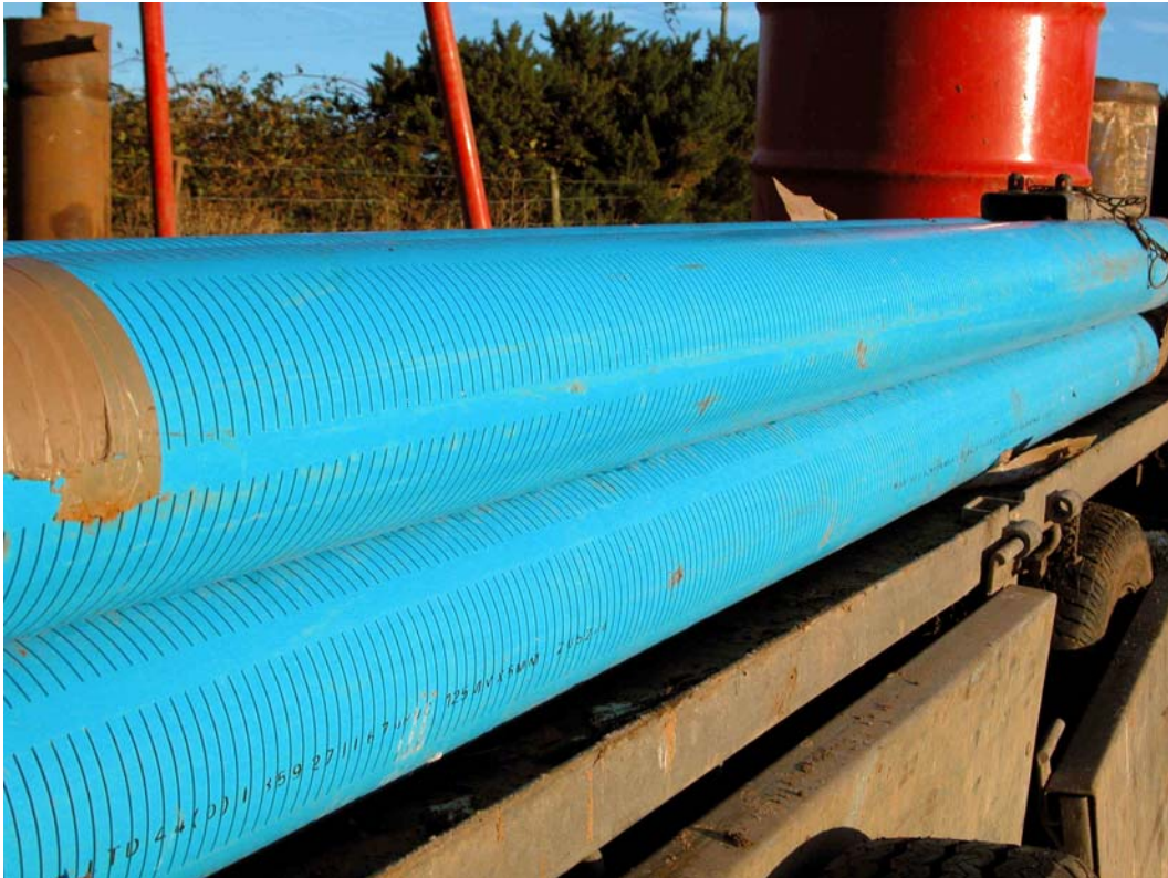
Figure 3 125 mm diameter plastic well screen was used in the boreholes
