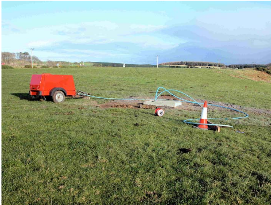
Figure 28 Whitecrook Farm borehole air-flush arrangement
