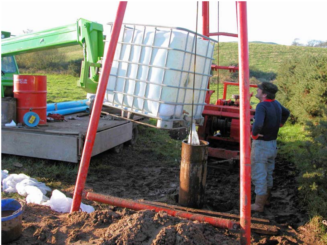
Figure 13 Adding water to aid the drilling process
