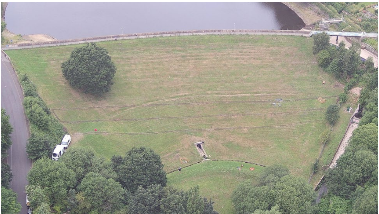
Figure 10 – Aerial view of the Dam
