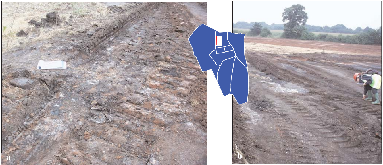
Figure 7.6 Stripped surface showing increased levels of Coal Measures mudstone, coal and brick fragments at NGR 451120 343000. The area was also identified as an area of soft ground.
