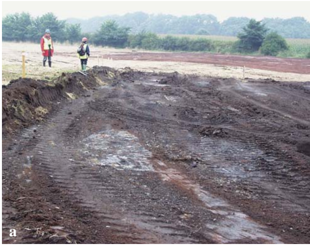
Figure 3.5 Evidence of mineshafts in the stripped soil at Chilwell Dam Farm.
