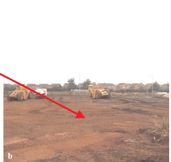
Figure 7.5 The effects of stripping on soil colour within the site; both images are of the same location.
