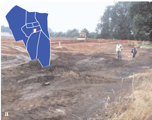
Figure 7.4a Soft ground at NGR 451255 342730 denoted by a series of ruts caused by the passage of site vehicles. Note the sharp boundary between 'clean' soil in the upper part of the image and darker, coal enriched soil in the foreground.
