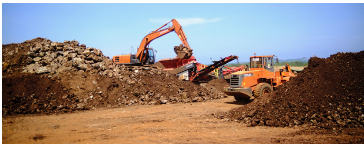
Nickel laterite ore processing through mobile crusher. Reproduced with permission from Nickel Asia Corporation.
