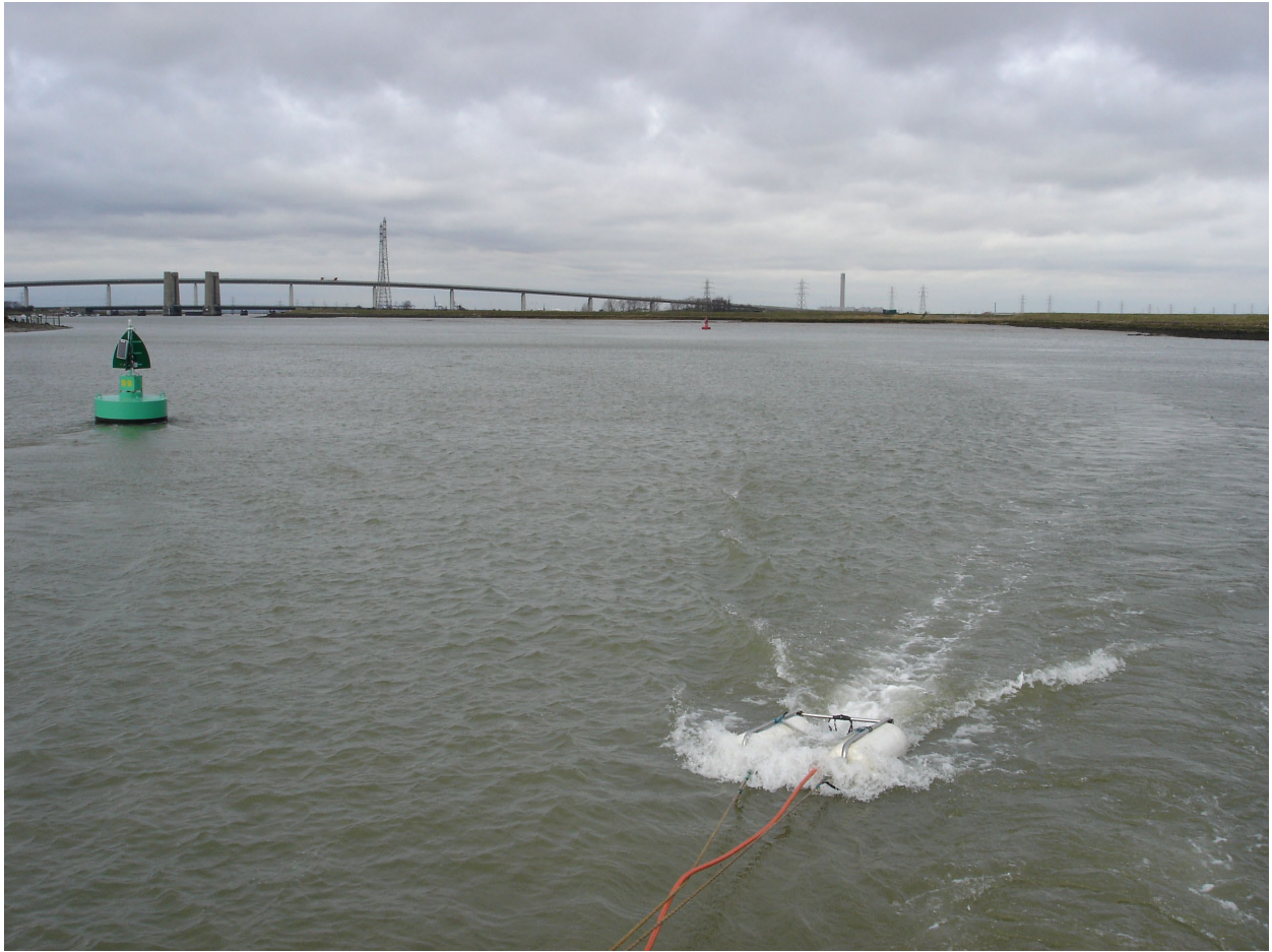
4. West end of Swale with Sheppey Crossing in background
