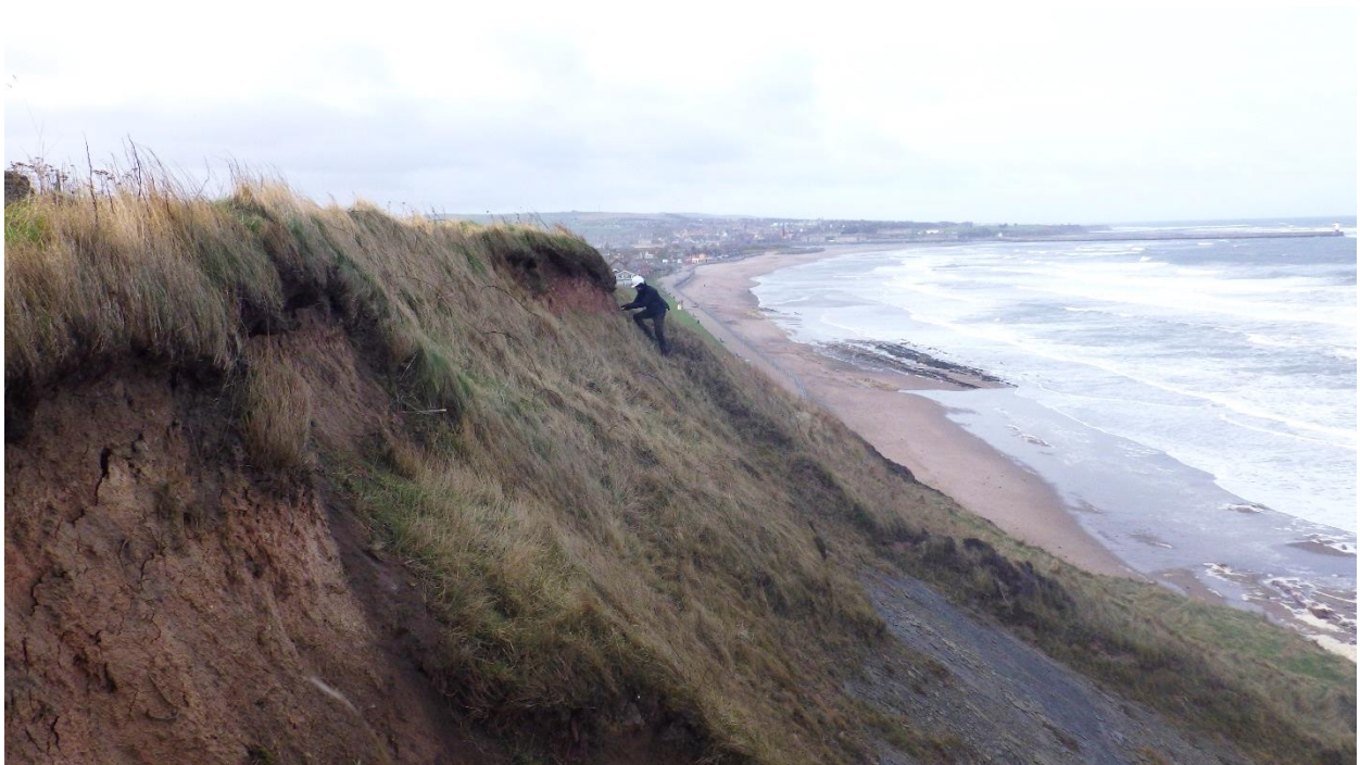
Figure 8 Head scarp of a minor landslide in till near the start of the coastal cliff section at the southern end of Spittal beach [401202, 650730]. The surface of a steeply dipping sandstone bed forms the dip slope seen in the bottom right of the image. Overlying till deposits have slipped on this bedrock surface but deposits have been largely eroded from the base of the cliff. View to the north. BGS image P1081720 © UKRI 2025.
