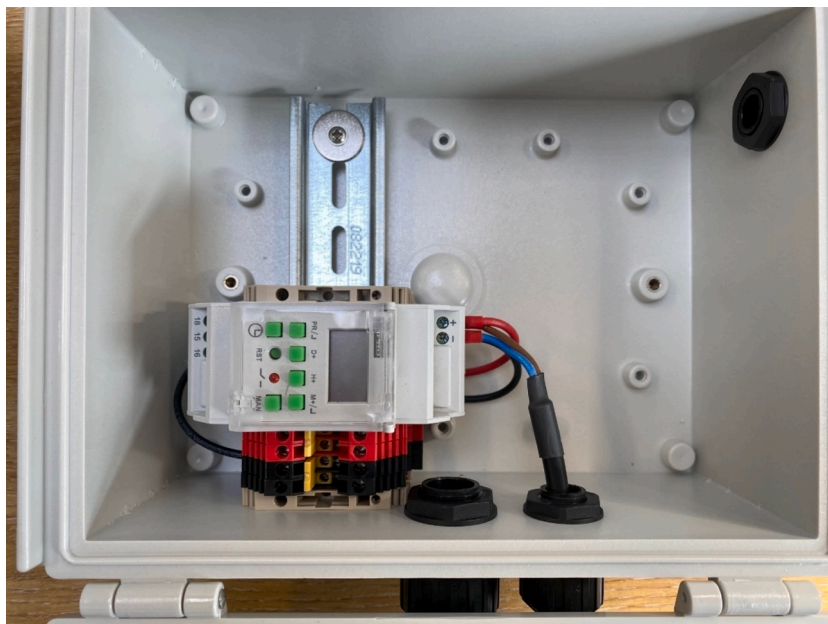
Fig. 7. Terminal block and timer relay installed on DIN rail (wiring described in later steps).
