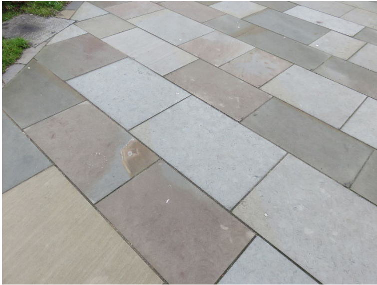
Above: Image showing an area of Locality 10's 'Island' in greater detail. The slabs with distinctly 'muted' colouration seen here are Whitworth Sandstone . The single slab-wide border (seen top left) is Caithness Flagstone .
