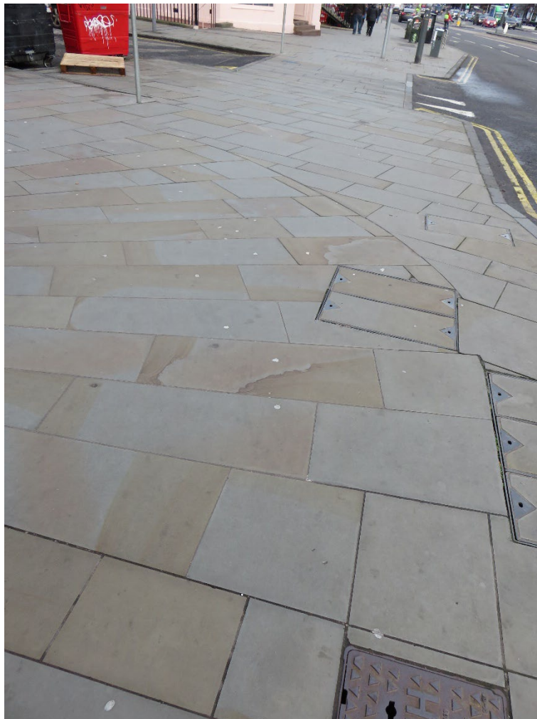
Above: Image, taken looking north-east, showing an area of the pavement located on the south-western corner of Union Street. Note the generally 'lively' colouration shown by the paving stone here, which is considered to be predominantly Scoutmoor Sandstone (sensu stricto) and/or Appleton Sandstone (pre-c. 2022 form). Stone with this appearance is prevalent within the stretches of pavement fronting Picardy Place itself (running between Broughton Street and Union Place) and Union Place (extending as far as the junction with seen in this image).
