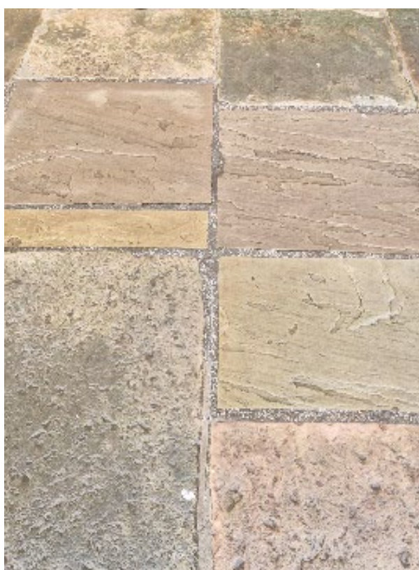
Above left: Stretch of Hailes Sandstone paving (as seen wet) present along the north side of Charlotte Square, illustrating the range of colours shown by this stone. Above right: Two rows of paving slabs located immediately outside the entrance to Bute House. Slabs of both Hailes Sandstone and a sandstone of probable Indian origin are present here; the latter are conspicuous owing to their colour and the distinctly different surface finish of the slabs.
