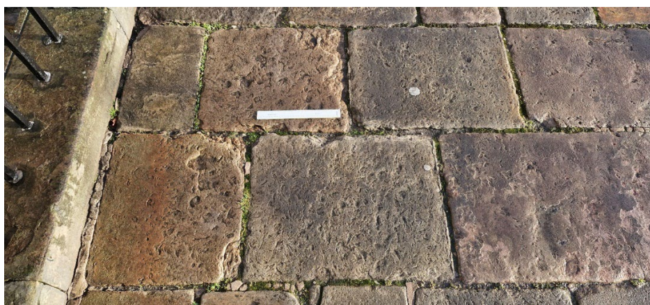
Above: Typical examples of Hailes Sandstone slabs observed at Locality 1, as seen wet; 30 cm ruler for scale.
