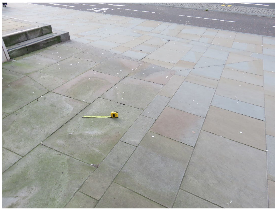
Above: Image showing an area of paving located immediately north of 'The Cube', on the south-east side of Leith Street. The interface between a small area comprising more weathered, apparently older (in terms of installation age), Scoutmoor Sandstone (sensu stricto) slabs and the typical, recently laid, Scoutmoor Sandstone (sensu stricto) paving of Locality 2 is well displayed. Weathering has picked out the irregular cross-lamination in the 'older' slabs, and as such their appearance is tending towards that of the historic Hailes Sandstone slabs of the New Town (not seen here). Tape measure (set at 30 cm) for scale.
