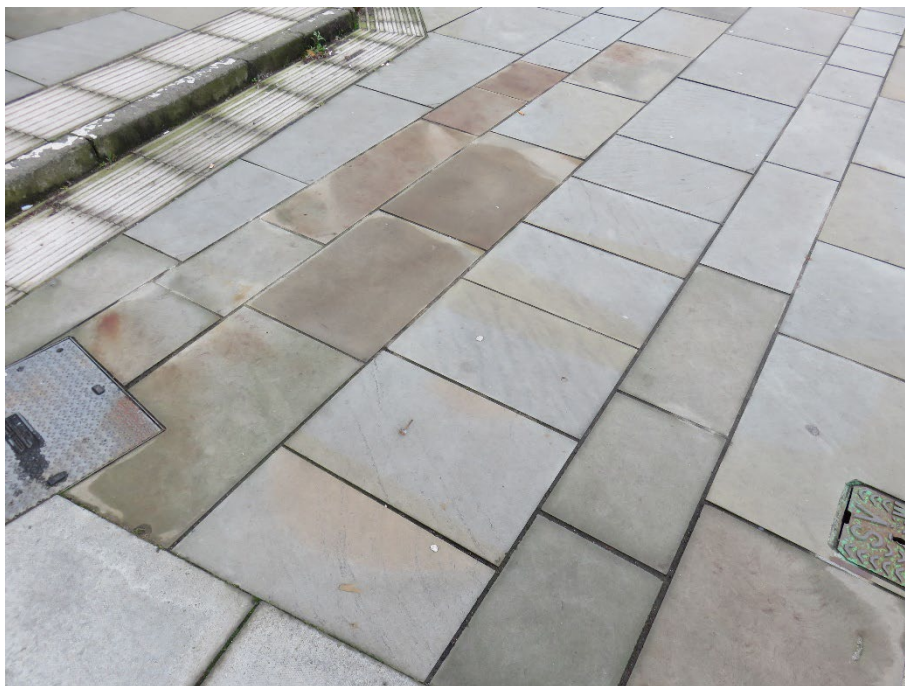
Above: Image showing an area of sandstone slabs (seen damp) forming the pavement at the Blenheim Place/London Road–Leith Walk junction. The slabs are variously 30, 45 and 60 cm wide. The discernibly higher proportion here of slabs showing more 'lively' coloration (something which becomes more pronounced as the pavement is followed south-westwards and Blaxter's Place is reached) is consistent with a greater presence of Scoutmoor Sandstone (sensu stricto) ± Appleton Sandstone .
