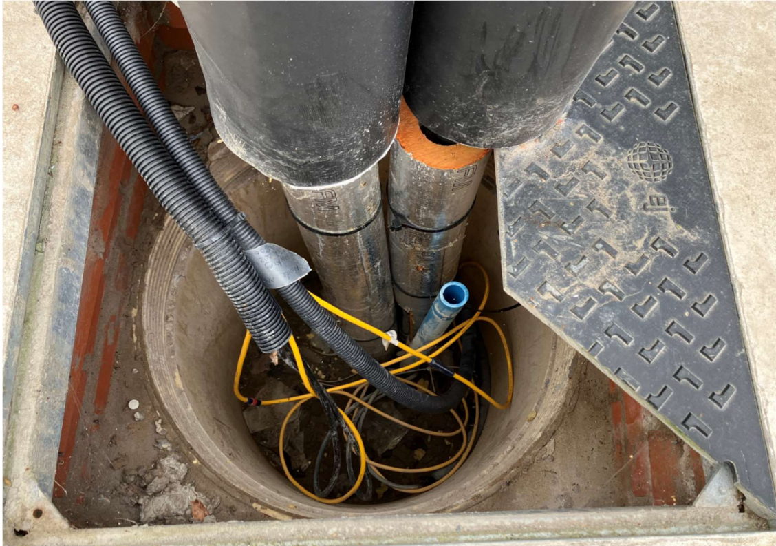
Figure 64 Wellhead chamber image TH0423
