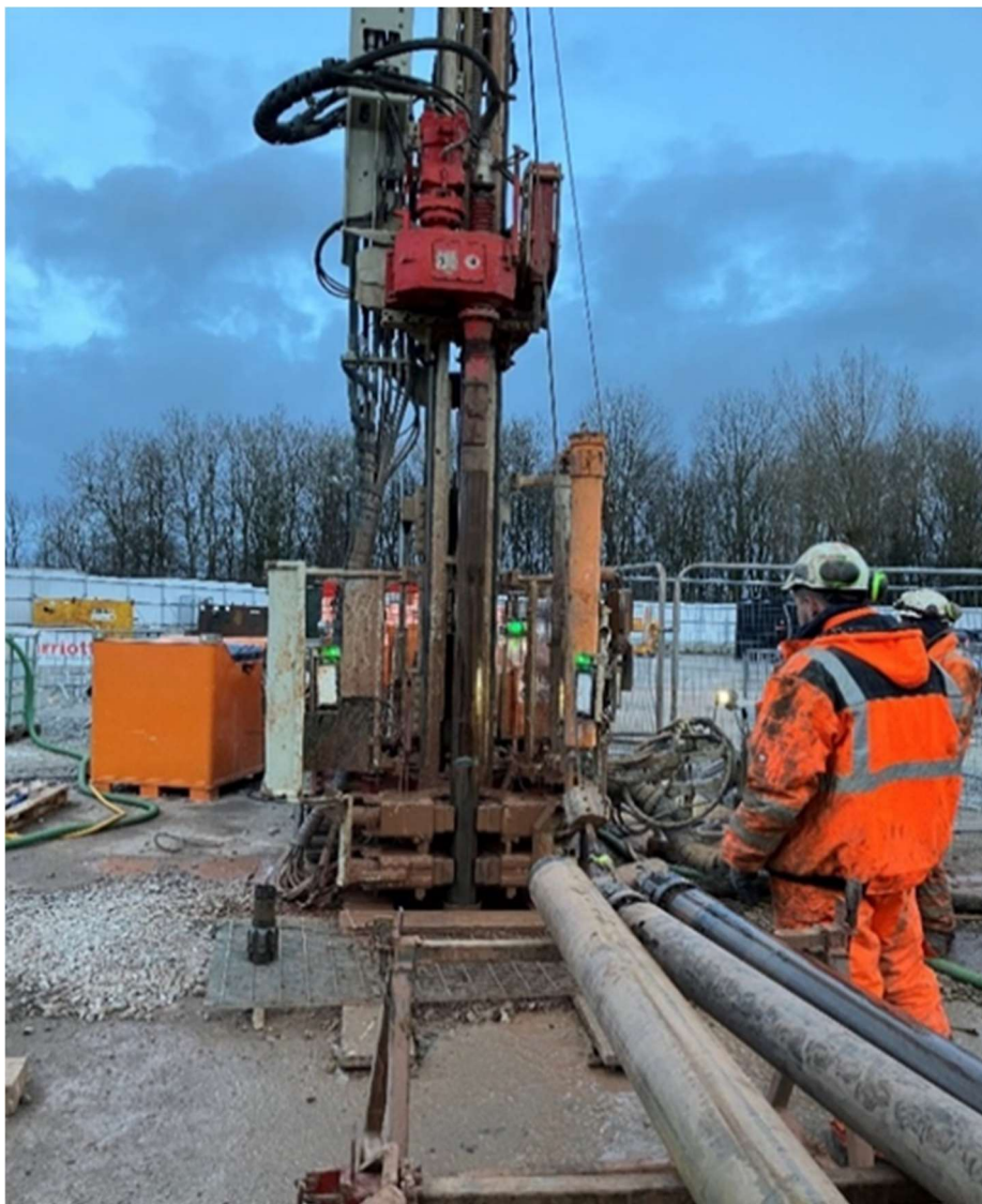
Figure 50 Coring ahead in TH0422
