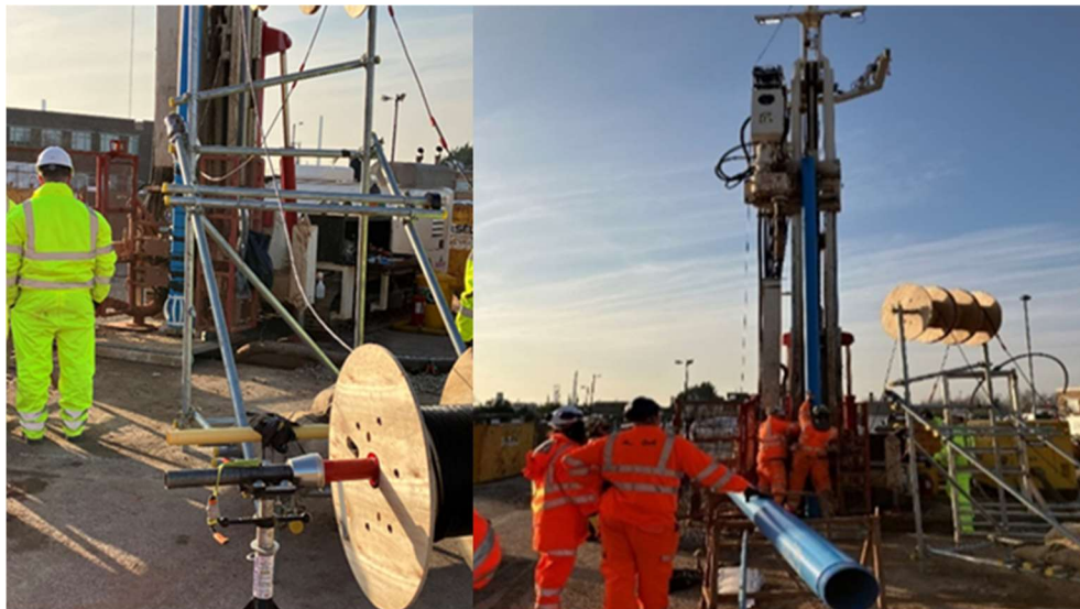
Figure 115 Installation of the 200 mm OD intermediate casing string
