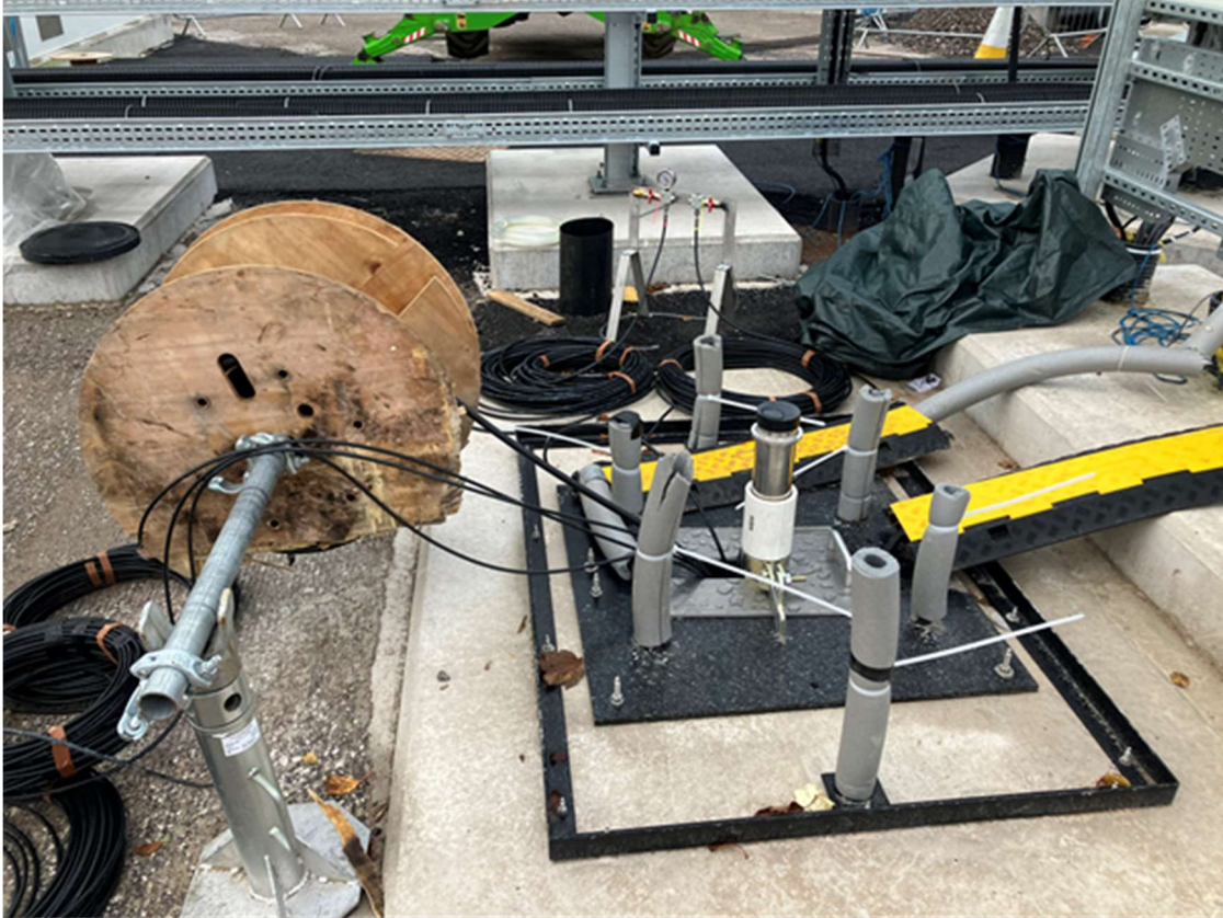
Figure 76 TH0408 pump and packer successfully RIH.
