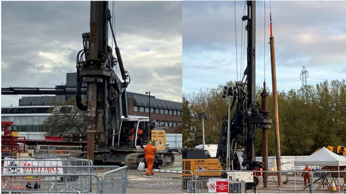
Figure 26 Marriotts Liebherr rig casing recovery operation
