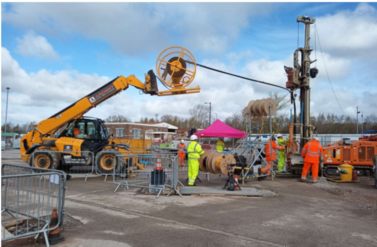
Figure 39 Image showing the Loop Master in operation as the installation is run.
