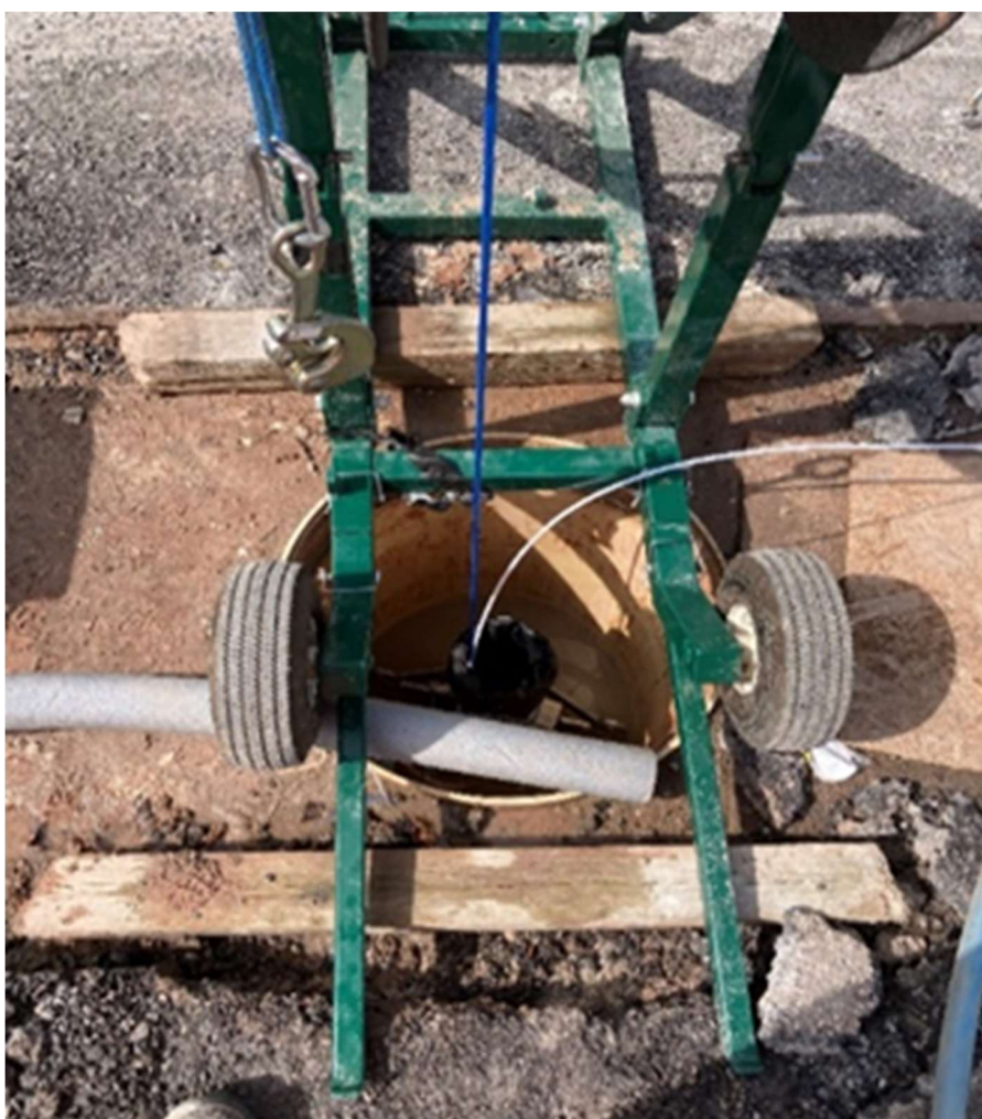
Figure 123 Green machine installed over the well during FLUTe liner deployment.
