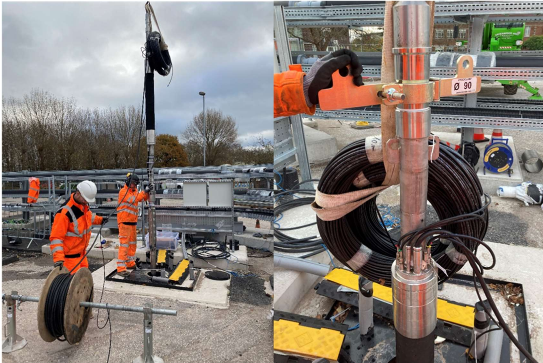
Figure 69 TH0406 pump and packer assembly being RIH
