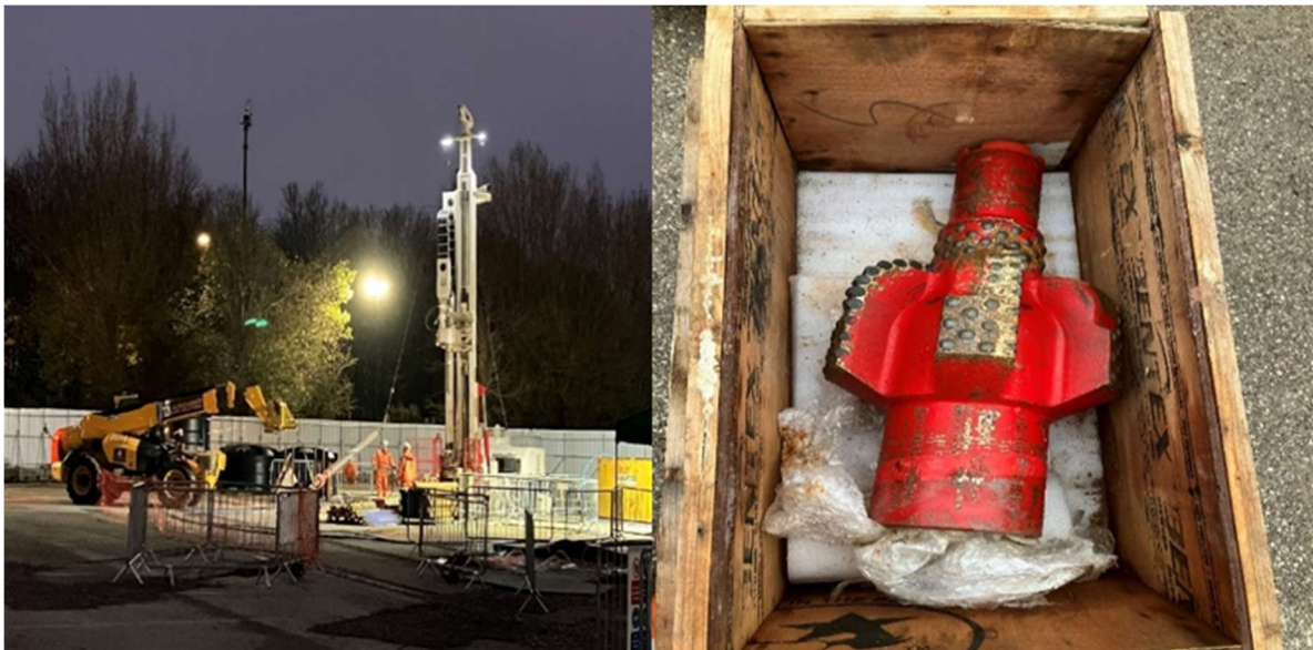
Figure 109 Lefthand image is of the 311 mm reamer assembly being picked up. The righthand image is the 311 mm reamer before make up
