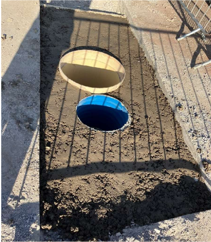
Figure 6 Installed 24” surface casing and smaller sump used during drilling phase only
