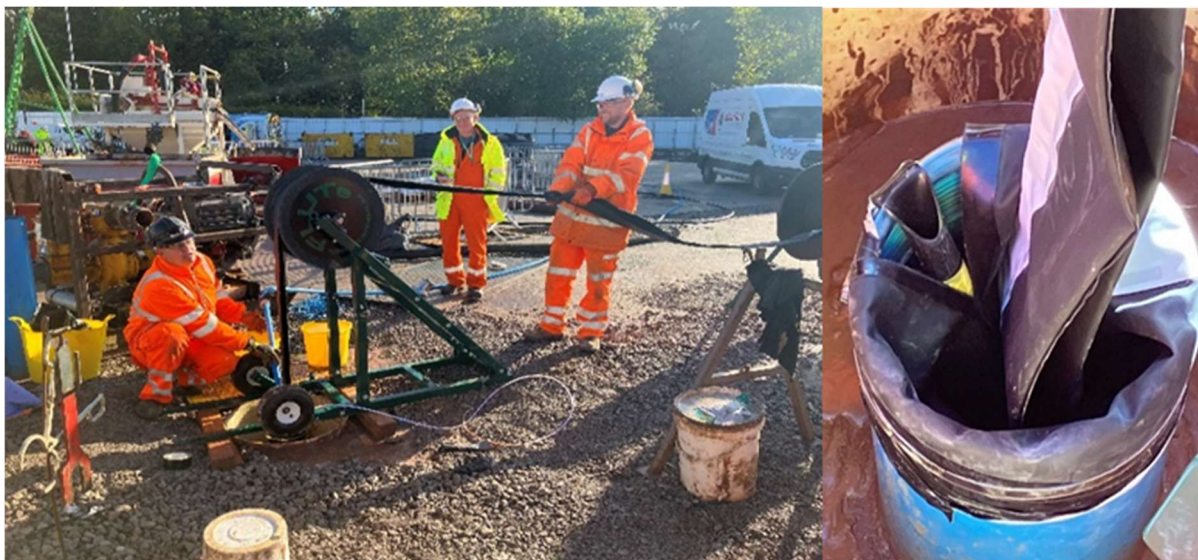
Figure 12 FLUTe liner deployment into TH0410 using “Green Machine”
