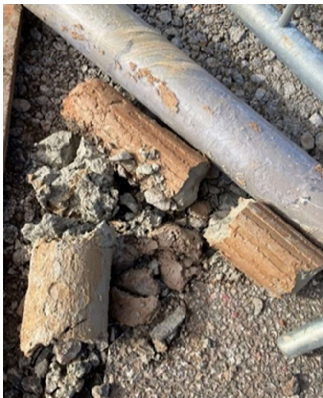
Figure 58 Cored out Geotherm X cement plug from 44.9 m to 47.9 m
