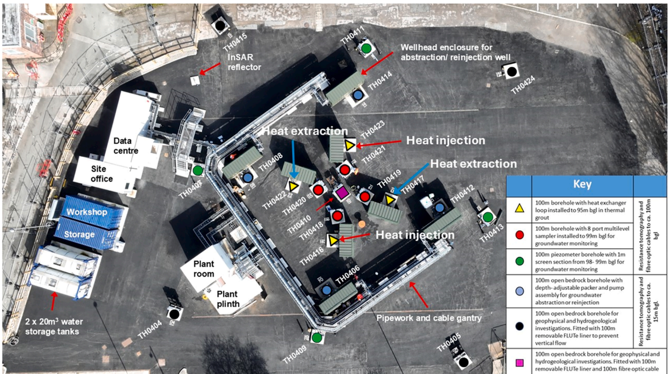
Fig. 2. Aerial photo of the site highlighting borehole locations. Note the yellow triangles are the 4 borehole heat exchangers used in the experimental set up. BGS © UKRI.
