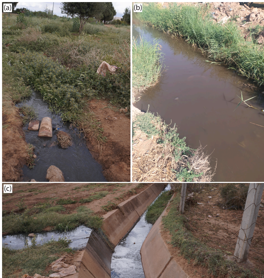
Fig. 2. Examples of wastewater management and reuse in the study area. Panels (a), (b), and (d) show direct discharging of untreated wastewater into traditional irrigation canals. These practices illustrate the potential for untreated effluents to enter recharge pathways and contaminate groundwater.
