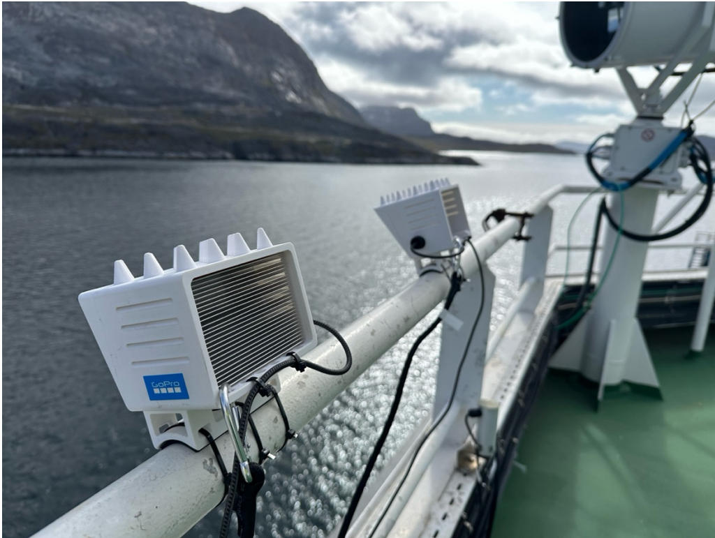
Figure 38: GoPro and Insta Ace Pro cameras and shrouds installed at Nuuk Harbour Greenland
