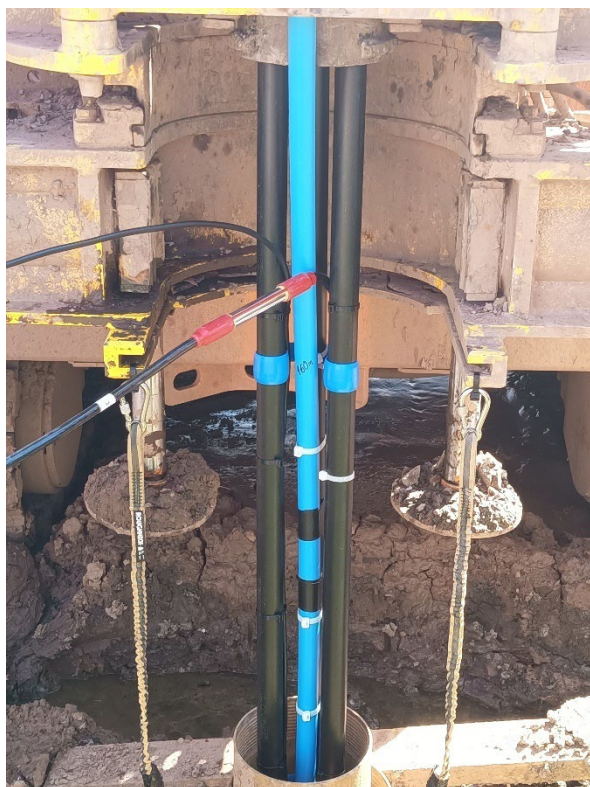
Figure 2: Photo of the 40 mm OD loop pipes and typical arrangement of sensor cables. The stainless-steel tubes with red end caps are ERT electrodes fixed to the ‘inflow to ground’ loop pipe, the black cable behind is the hybrid fibre optical cable tied onto the ‘return from ground/production’ side of the loop pipe. The blue 32mm pipe is a ~100 m long shallow tremie and the black 32mm pipe behind it is the ~210 m long deep tremie. The blue clip is
