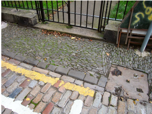
Photo 59. Entrance to central gardens area, Moray Place, showing whinstone horonized pavement with perpendicular pattern adjacent to the entrance, with whinstone setted kerb, and granite setted gutter and road surface. An original sandstone lighting plinth is preserved to the right-hand side of the entrance.
