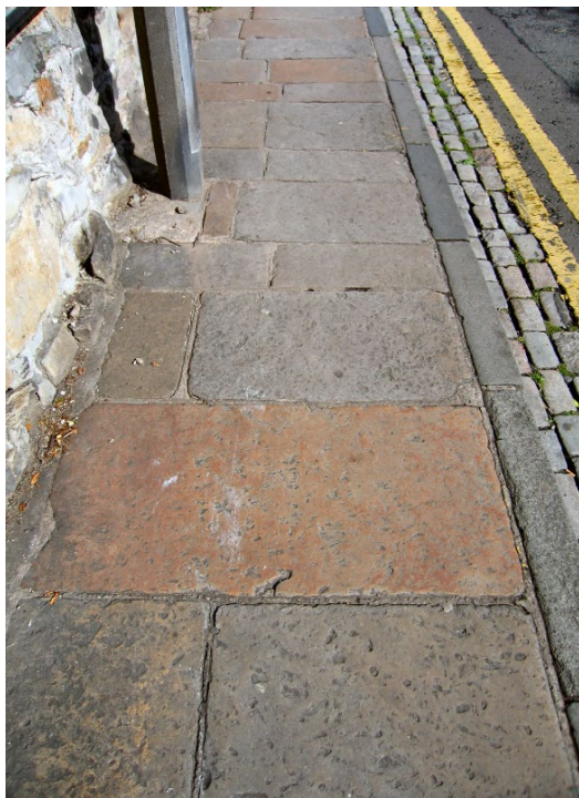
Photo 9. Traditional sandstone paving showing the typical range of colours and natural surface textures caused by presence of ripple bedding within the sandstone. This provides a natural anti-slip surface (Bell's Brae).
