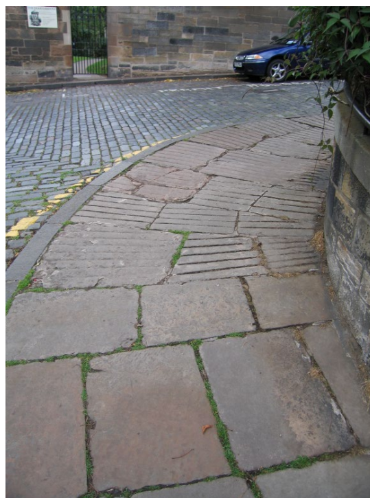
Photo 5. Corner of Ann Street and Upper Dean Terrace with slabs showing tooling with parallel grooves cut as an anti-slip measure on the slope. Note the course width fan-out around the corner.
