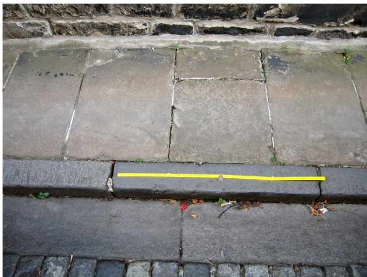
Photo 41. Gloucester Lane pavement showing sandstone slabs, whinstone kerb, dished whinstone gutter stone and setted road surface. Scale is 1 metre long.
