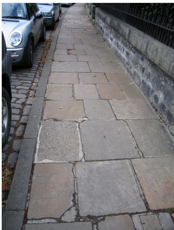
Photo 3. Typical section of sandstone paving in Ann Street showing relatively small slab size and range of colours from grey to reddish-brown. Note the variable surface texture including ripple textured surface to some blocks.
