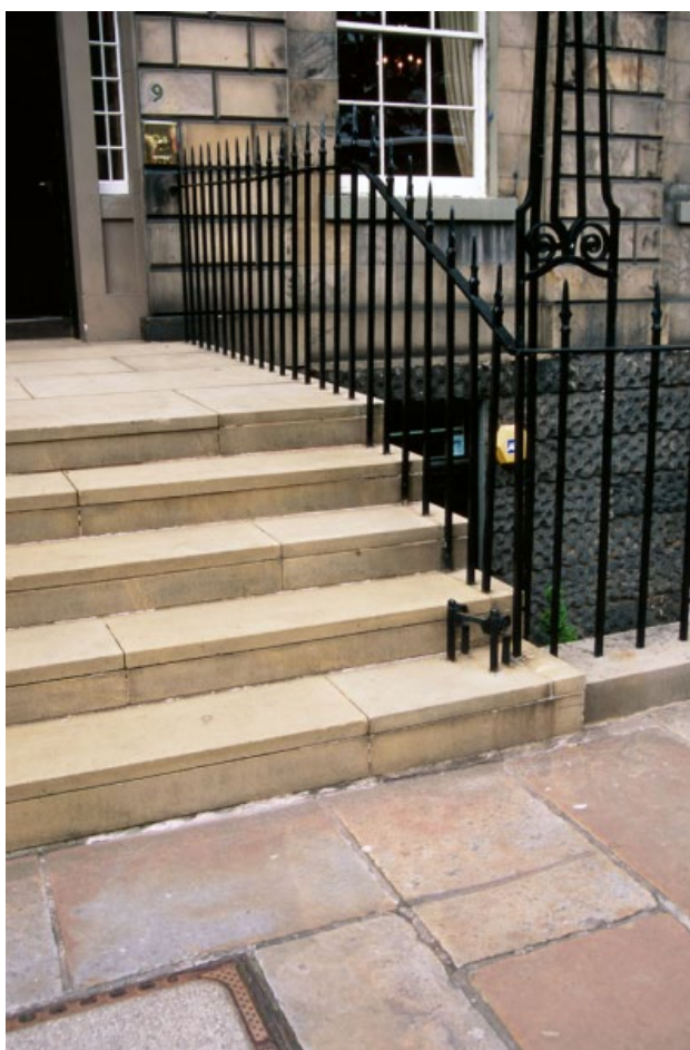
Photo 77. Use of replacement Yorkshire sandstone as replacement steps adjacent to original 'Hailes type' sandstone paving. The typical uniform yellow-buff colour of the York stone contrast with the more variable and stronger coloured original paving slabs.
