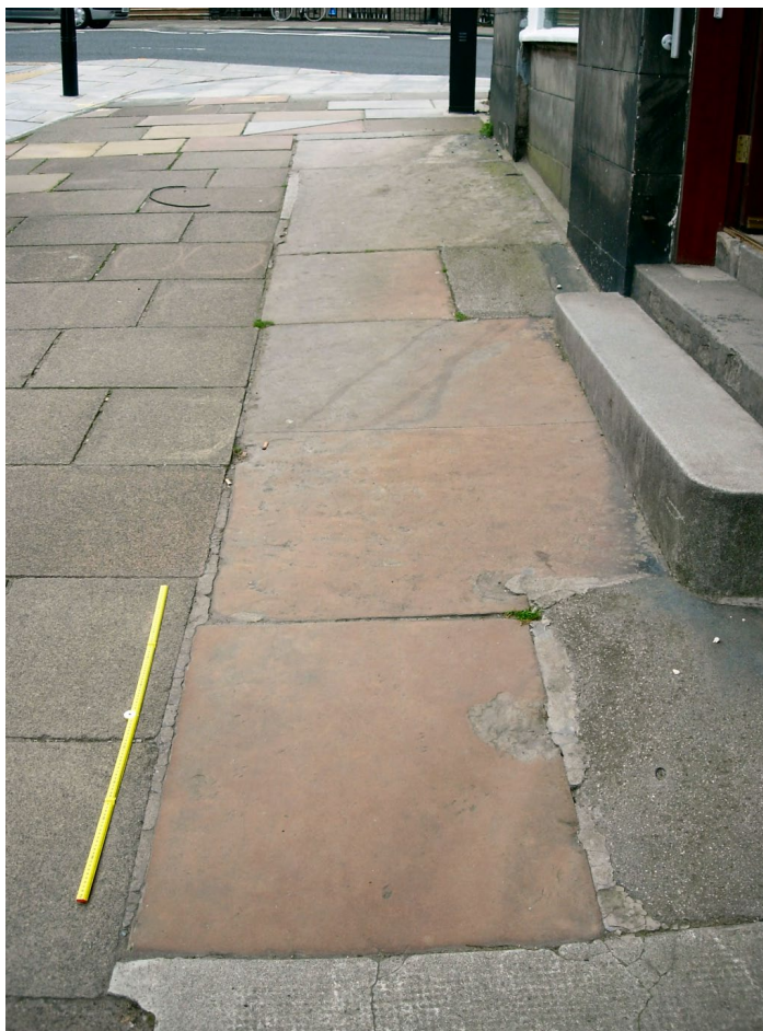
Photo 45. Remains of original stone paving in Wemyss Place with large slabs of characteristic orange-brown weathering sandstone, with replacement concrete slab over most of the pavement. The steps to the adjacent property entrance are also sandstone.
