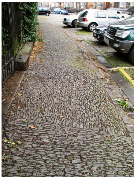
Photo 60. Typical whinstone horonized pavement with perpendicular pattern adjacent to garden entrance, with whinstone setted kerb, and granite setted gutter and road surface. Northwest garden entrance, Moray Place.
