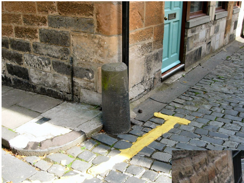
Photo 24. Whinstone spur stone Carlton Terrace Mews, with whinstone setted roadway and dished gutter stones.
