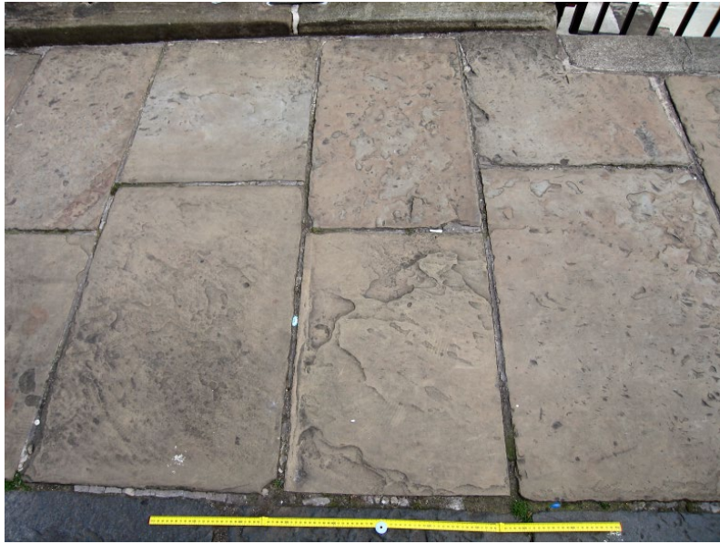
Photo 51. Detail of original paving in St Stephen Place showing typical variation in colour and surface texture and uniform offset laying arrangement.
