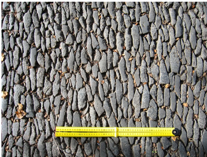
Photo 54. Horonizing in Glenfinlas Street, showing typical well packed dolerite (whinstone) fragments. Scale ruler 50cm long.
