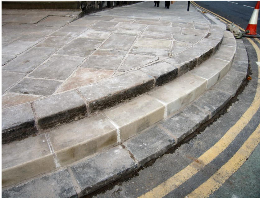
Photo 47. Recently repaired and re-laid original sandstone paving and kerb at the northeast corner of Charlotte Square, reinstating the previous paving arrangement following disruption from repeated service works over many years. Because of damage to some original kerb stones, the middle row of kerb steps has been replaced using a sandstone from the north of England. The standard of workmanship and the care taken to reuse original materials where possible should be seen as a model of good practice. The photo was taken immediately after completion of the work before the area had been cleaned to remove excess sand and mortar.
