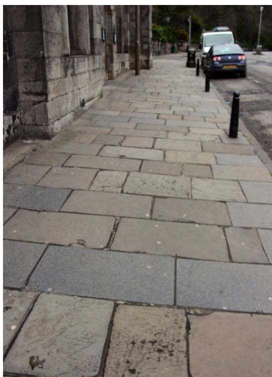
Photo 31. Re-laid sandstone paving in Waterloo Place, showing a mixture of original sandstone blocks which have been redressed to smaller uniform sizes, interspersed with Caithness flagstone (dark blue-grey slabs) and modern York sandstone paving (uniform buff-grey colour). The original sandstone flags have a more variable colour and variable surface texture.
