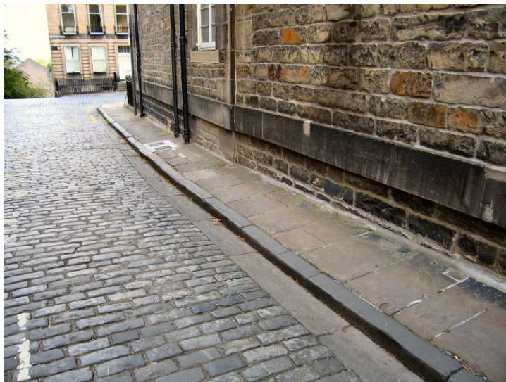
Photo 40. Entrance to Gloucester Lane showing typical arrangement of a single row of sandstone slabs aligned perpendicular to the kerb, with whinstone kerb, dished gutter and setted road surface. The pavement surface is a grey-brown sandstone with a reddish-brown patina on worn surfaces.
