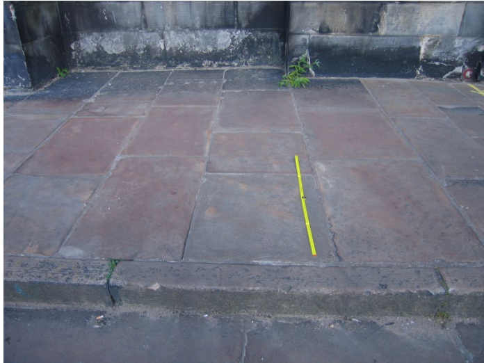
Photo 28. Detail of sandstone paving in Regent Road showing the courses aligned perpendicular to the kerb, with long kerbstones and gutter stones both made from similar sandstone. Note the dark discoloured surface where the slabs are less worn along the inside of the pavement -here the original broached tooled surface of the sandstone is preserved. Scale is 1 metre long.
