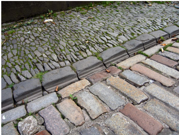
Photo 57. Whinstone horonized pavement in Ainslie Place, with whinstone kerb and granite gutter and setted road surface. Note the wear to the kerb stones.
