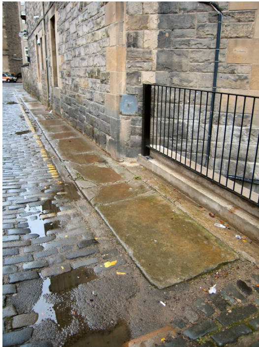
Photo 11. Typical single width sandstone paving in a lane, with large slabs aligned parallel to the lane, and no kerbstone. Note the poor maintenance of the whinstone setted lane. (Lynedoch Place Lane).
