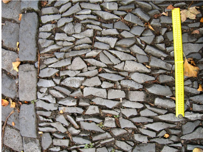
Photo 55. Horonizing on St Colme Street showing irregular sized whinstone fragments, noticeably less well packed than that on Glenfinlas Street. The kerb is formed from a single line of whinstone setts. Scale rule is 50cm long
