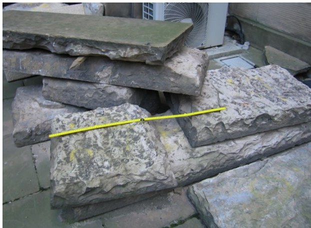
Photo 38. Lifted (and mostly overturned) paving slabs from the basement area on the east side of General Register House. The unworn underside surfaces show the characteristic irregular ripple bedding defined by dark carbonaceous layers, typical of Hailes sandstone. Note the uppermost slab, which is the correct way up, shows a typically smooth worn surface which is darker in colour with traces of ripple bedding.
