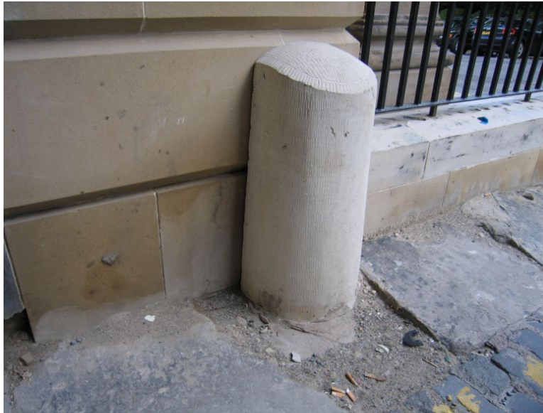
Photo 44. Recently reinstated replacement sandstone spur stone at entrance to Wemyss Place Mews.
