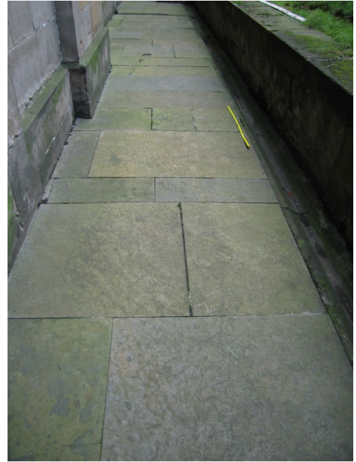
Photo 37. 'Historic' Caithness flagstone paving surrounding New Register House, showing variable dark colours with a distinctive dark 'flecked' surface texture typical of this stone type.
