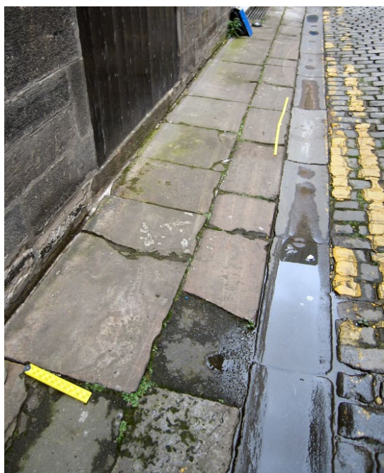
Photo 16. Thistle Street NE Lane. Single row of sandstone flags aligned parallel to the broad sandstone kerb, with dished whinstone gutter and whin setted roadway. Note tarmac repairs to broken and missing kerbstone.
