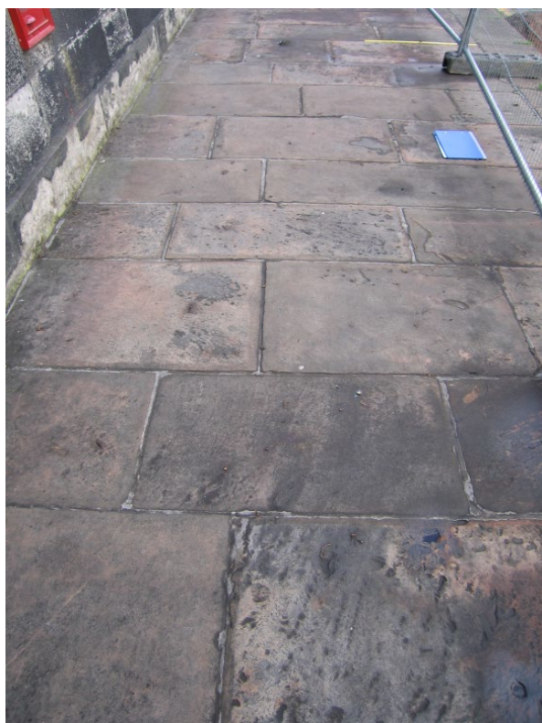
Photo 26. Sandstone pavement in Regent Terrace, showing relatively regular-sized and uniform large blocks with typical dark grey-buff colour with a reddish brown patina on worn surfaces. The variable, naturally rough surface is caused by the ripple bedded nature of the sandstone.
