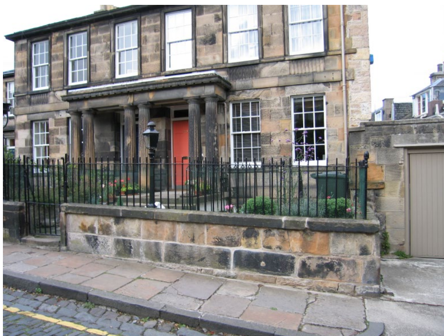
Photo 6. Traditional stone materials with whinstone roadway (setted street, gutter and kerbs) and sandstone flags to pavement, with sandstone boundary walls and buildings. The preservation of natural stone materials provides a continuity between the streetscape and buildings. (Ann Street).
