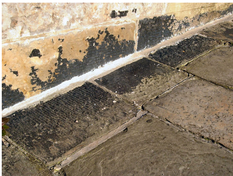
Photo 49. Sandstone paving in Glenfinlas Street, showing original broad broached tooling preserved in the less-worn areas adjacent to the inner boundary wall. The paving shows the typical variation in colour and texture characteristic of original sandstone paving in Edinburgh.
