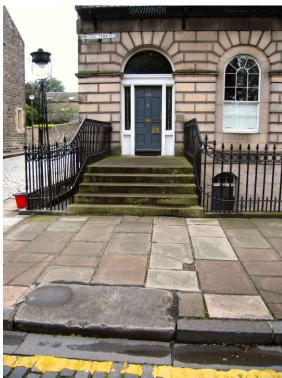
Photo 22. Original sandstone kerb block at the pavement edge (large grey block), directly opposite a property entrance, with whinstone kerbs, dished whinstone gutters and setted roadway. The pavement itself has been re-laid with coloured concrete slabs.
