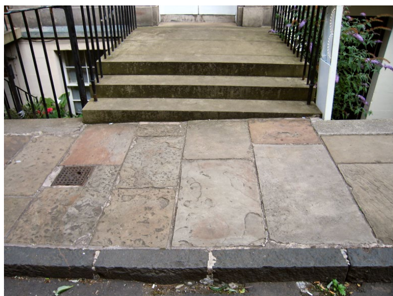
Photo 50. Sandstone paving in St Stephen Place showing typical variable appearance and surface textures, with colour ranging from grey to reddish-brown. The steps and entrance plat are replacement 'York sandstone' rebuilt in 1985.
