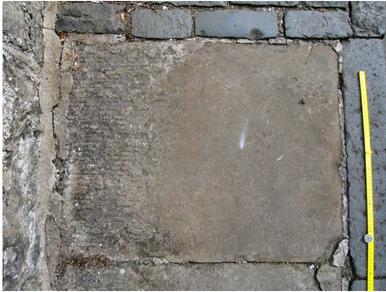
Photo 42. Detail of sandstone paving slab in Gloucester Lane showing typical brownish-grey colour and fine to medium grained texture, with remains of original broached tooled surface preserved where less worn close to the wall (left-hand side). Ruler scale is c.750 mm long.
