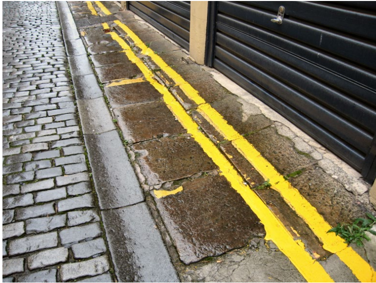
Photo 19. Well-preserved section of sandstone paving in Young Street N Lane, showing a double row of sandstone flags aligned parallel to the kerb, with dished whinstone gutter and whinstone setted roadway.
