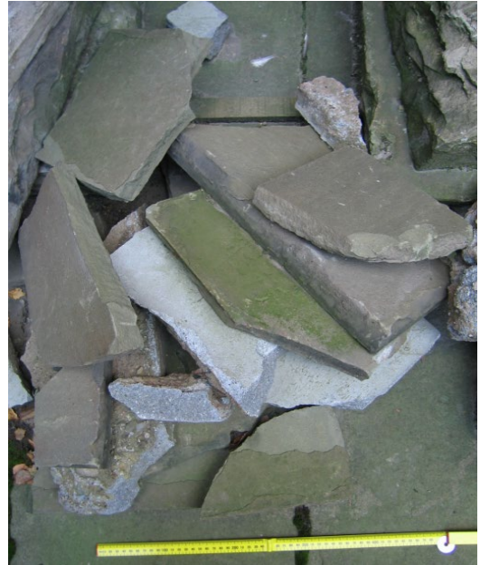
Photo 39. Lifted and broken paving slabs from basement level at the rear (north) side of General Register House, showing dark purplish-grey-green colour with a fine grained uniform texture. These features are characteristic of Carmyllie flagstone.
