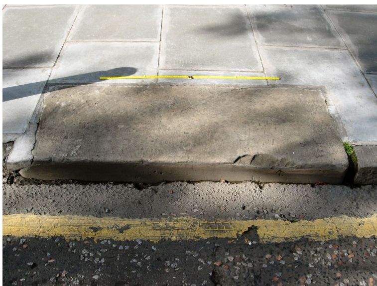
Photo 15. Large sandstone mounting block opposite a property entrance in Coates Crescent (No. 16). A number of these original mounting blocks are still present, although all the pavement surfaces have been replaced by concrete.
