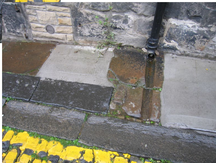
Photo 21. Poorly preserved area of original sandstone paving with carved drainage channel in sandstone below the downpipe outfall. Note the light coloured cement patch repairs (Young Street S Lane, west return to Young Street).
