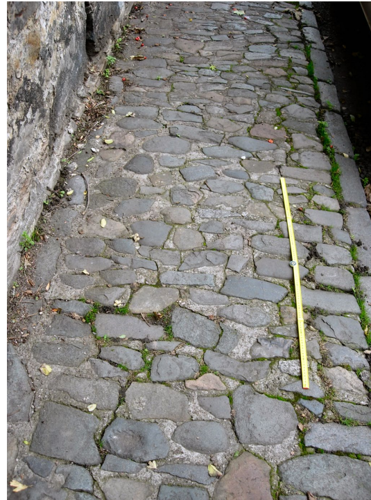
Photo 8. Pavement on Dean Path constructed using a mixture of cobbles of different stone types and reclaimed whinstone setts.
