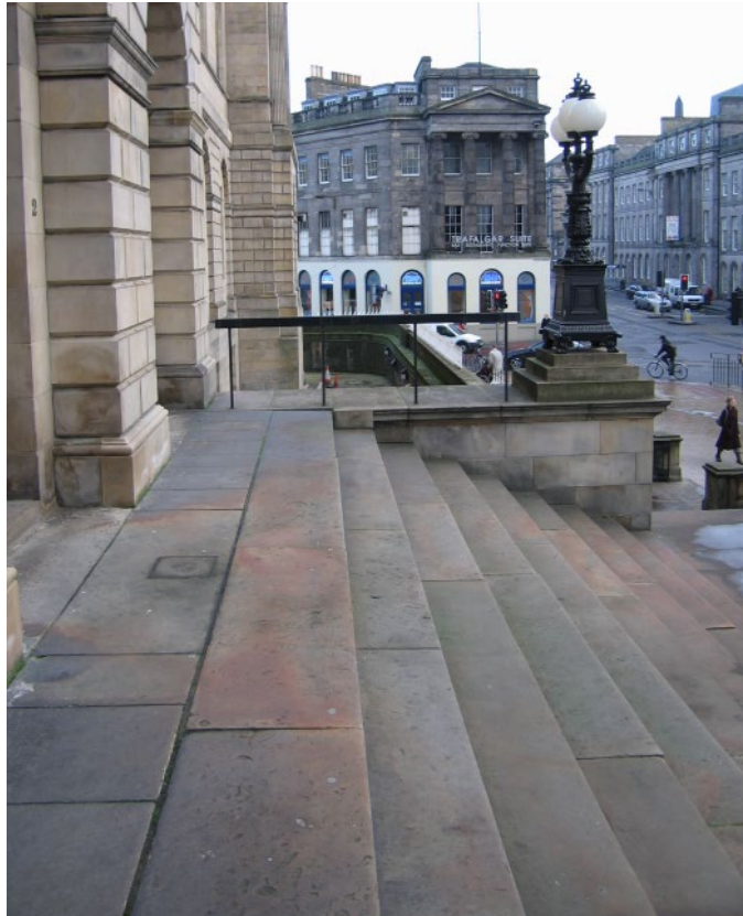
Photo 35. Main entrance steps, General Register House, showing characteristic greyish-brown colour with reddish-brown patina on worn surfaces.
