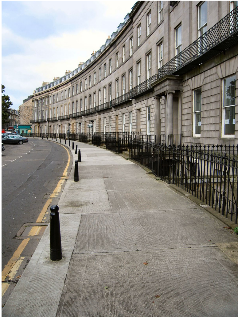
Photo 14. View of Atholl Crescent showing the presence of unsightly concrete pavement. A number of entrances to coal cellars are present at the road edge, marked with sandstone surrounds.
