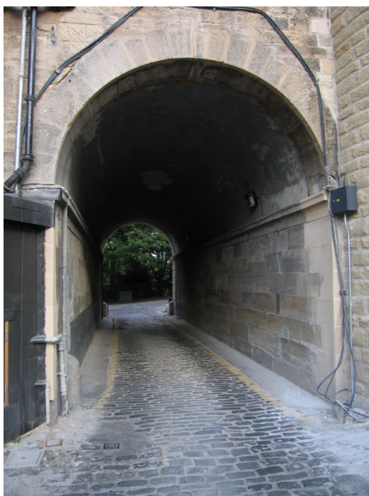
Photo 43. Recently refurbished covered lane entrance to Wemyss Place Mews, with original sandstone pavement and setted roadway. Spur stones are present on three of the four corners.
