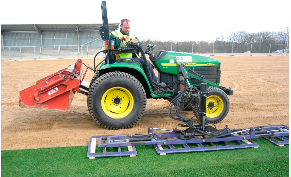
Sand used in sports pitch construction. © Holcim UK
