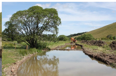
2013 July - cutting the new channel
