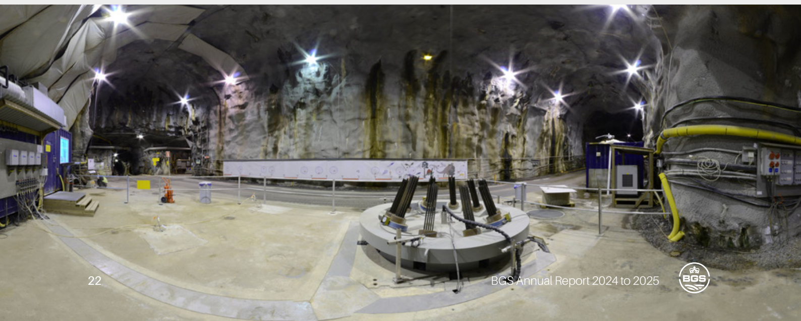
Figure 12 The surface infrastructure of the Large Scale Gas Injection Experiment (Lasgit), operated 800 m underground in the Äspö Hard Rock laboratory. BGS © UKRI.
