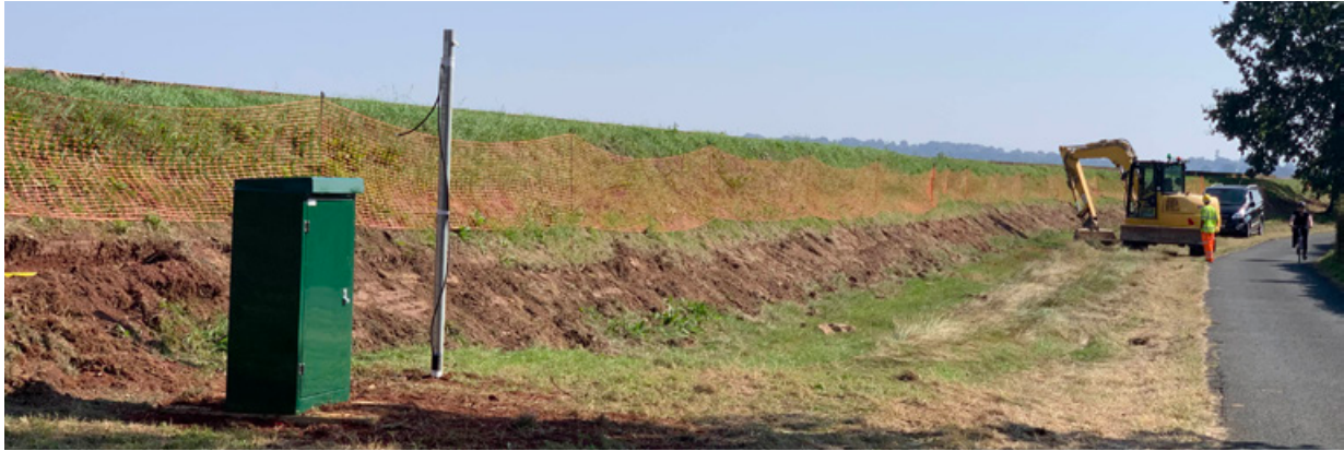
Figure 20 View along the Powderham Banks flood embankment on the Exe Estuary, Devon. This historic structure, now monitored by BGS's PRIME technology, plays a critical role in protecting key transport links and local communities from flooding. BGS © UKRI.
