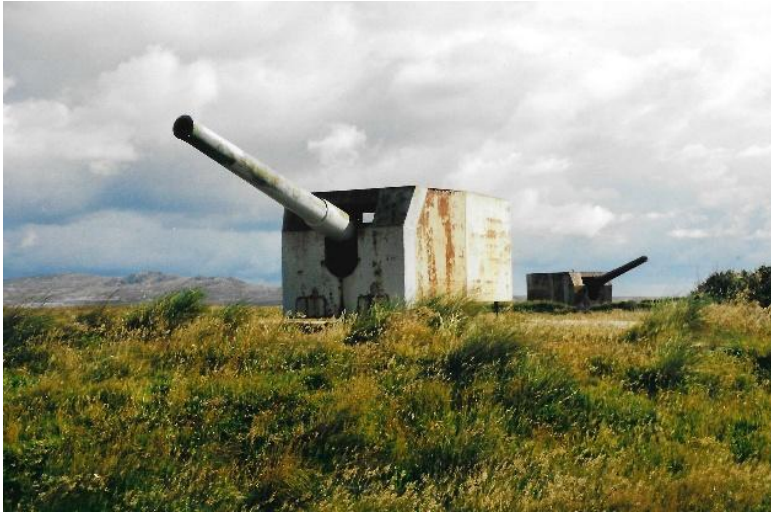
Figure 4. The six-inch Naval guns installed on Canopus Hill in the 1930s and 1940s. Reputedly, 22 feet (6.7 m) of peat had to be removed to establish the foundations (Penguin News, February 25, 2005, 10-11). This photograph was taken in 2001; the guns were repainted in 2005. British Geological Survey image P1074033 © UKRI 2001.
