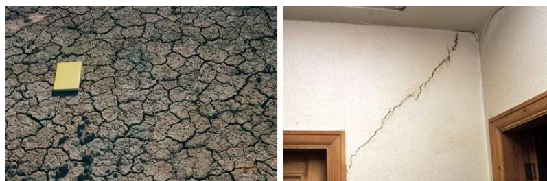
Figure 27 a (left) shrinkage cracks in Lambeth Group clay; b (right) subsidence caused by shrink/swell.
