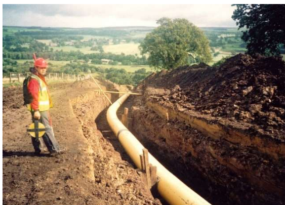
Figure 18 High pressure gas main investigation at Ben Rhydding, W. Yorkshire (2001).
