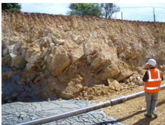
Figure 19 Horizontal directional drilling at Hailes Bank, Wormington to Sapperton pipeline route (2010).
