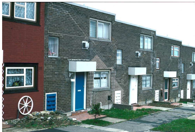
Figure 26 Terrace of houses on London Clay in Essex showing the differential settlement as the terrace crosses a hedge line.
