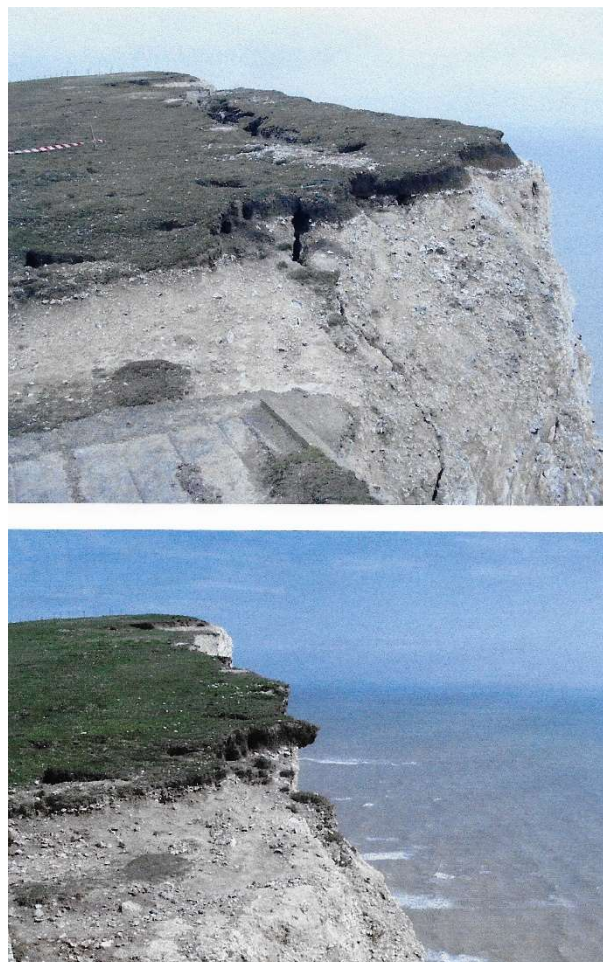
Figure 20 Pre- and post- rock slide of 8 April 1999 at Beachy Head.
