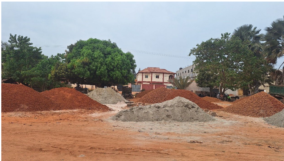
Figure 4 Kololi Tipper Garage, crushed laterite in the background and marine sand in the foreground
