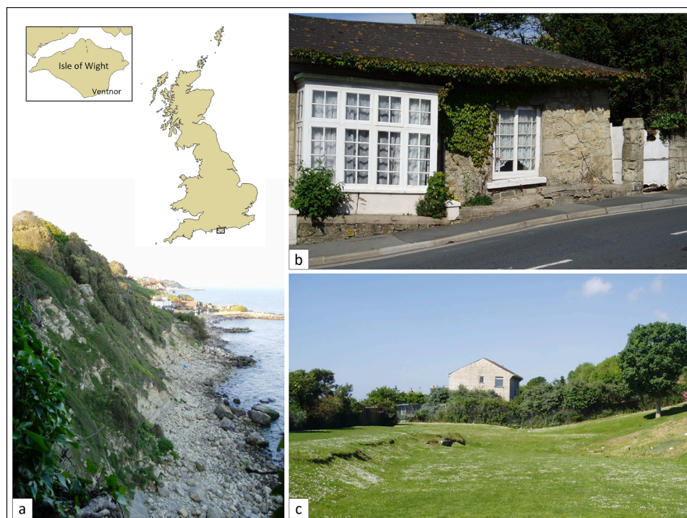
Fig. 10. Ventnor, Isle of Wight, case study; a) Toe of the Undercliff; b) Property damage; c) Ventnor Graben ( http://geoscenic.bgs.ac.uk/ ).
