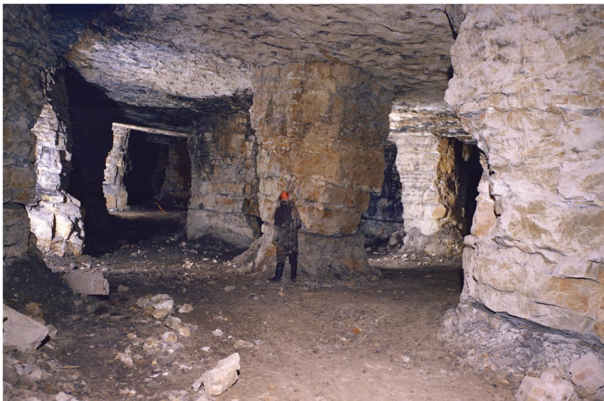
Plate 8 Blackhall Limestone, Lower Limestone Formation; Middleton Quarry [NT 3530 5750]; underground view showing dimensions of stoops and rooms, lowest 6 m of 15 m thick seam extracted (P001518) BGS © UKRI
