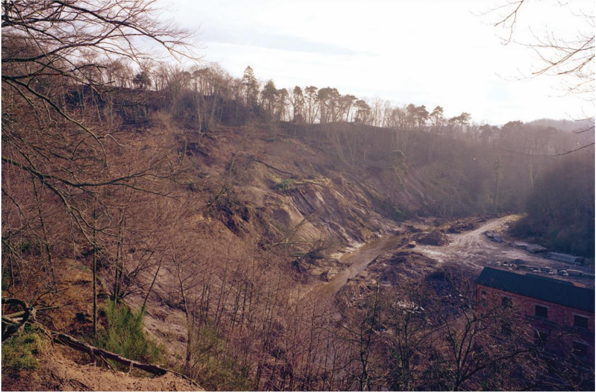
Plate 16 Springfield Mill, west bank of River North Esk, Polton Bank [NT 2850 6468] View of 1980 landslide looking south-south-west, showing 10–15 m. high foot scarp and numerous subsidiary scarp features up slope. Landslide toe (removed) formerly extended across River Esk almost to left-hand edge of photograph, between tall brick building (lower left) and wire fence behind (P219748) BGS © UKRI
