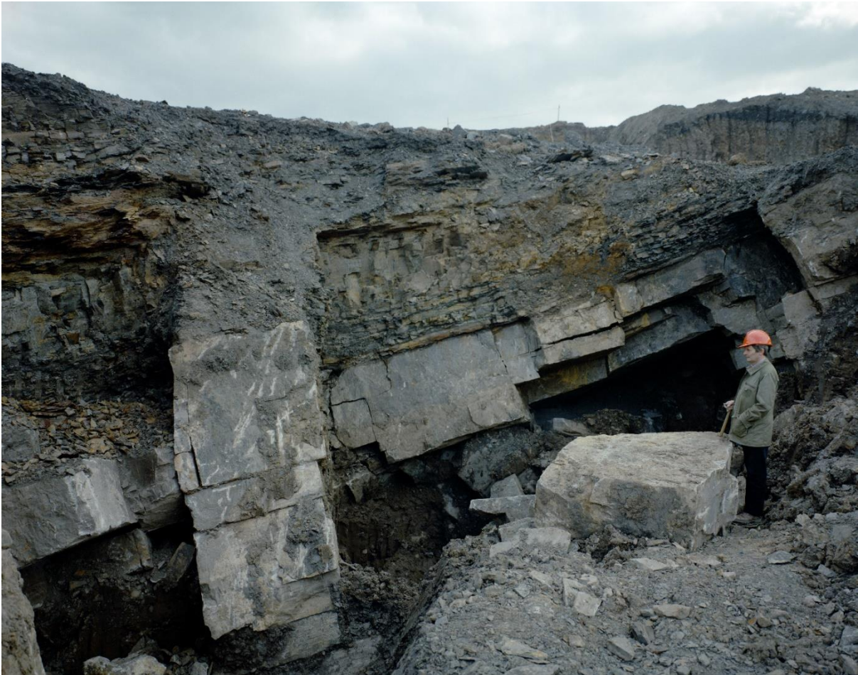
Plate 7 Burdiehouse Limestone; stoop and room mineworkings in excavations for the Edinburgh City Bypass [NT 2750 6690]; detail of roof and support pillars with overlying mudstone strata, void space partly filled with glacial till from collapsed crown holes nearby. (P220286) BGS © UKRI
