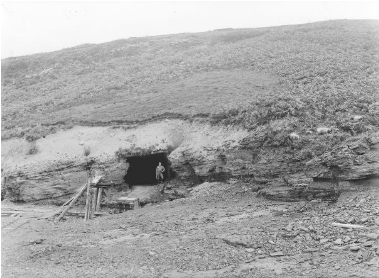
Fig. 12.9: The Raasay Ironstone Mine. 1.6 km east of Raasay House, Island of Raasay. Trial adit from Mine No. 1 driven through the Lower Jurassic Scalpay Sandstone into Portree Shale and ironstone, dipping WNW. BGS photo P000039 taken in 1917. [BGS © UKRI].
