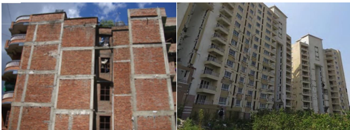
(Group, Seismic Vulnerability Assessment Project, 2013)
