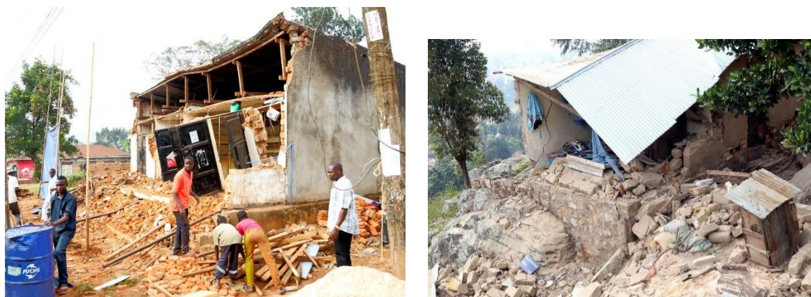
Figure 4.2: Brick Masonry (left) and adobe mud block (right) building which suffered complete damage during the 2016 earthquake (AFP 2011).
