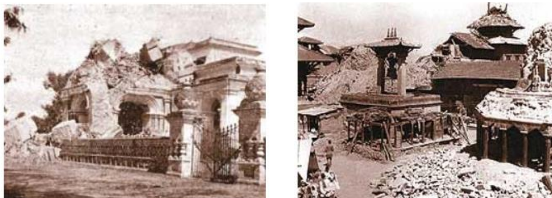
Figure 3.4: Collapsed buildings during the 1934 earthquake in Nepal (source: Nepalese Times).
