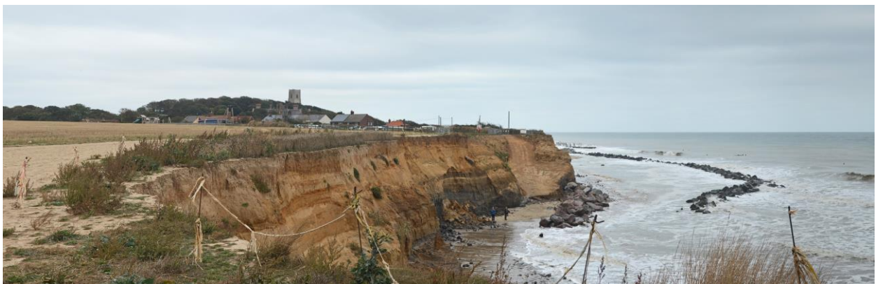
Figure 2: Cliff erosion evident at Happisburgh, Norfolk
