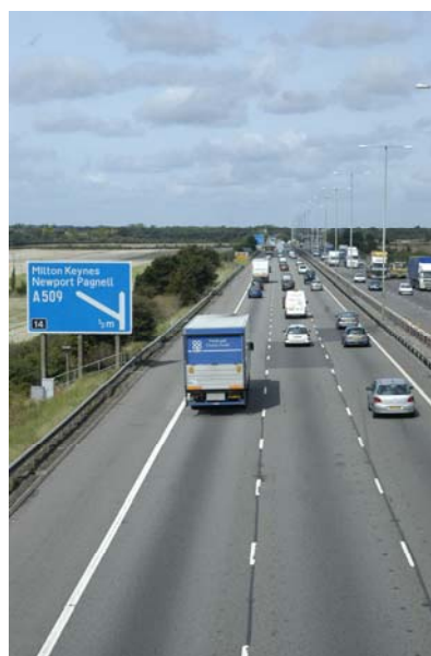
Plate 5 The first section of the M1 was built in the Project Area in 1958/9
