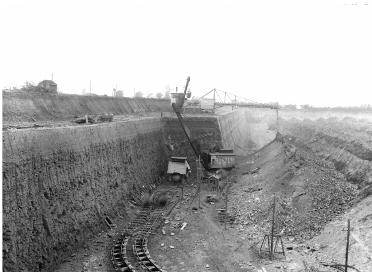
Plate 3 Extraction of Oxford clay at Beeby’s L.B. Pit, Fletton, for the brickmaking industry of the 1940s.
