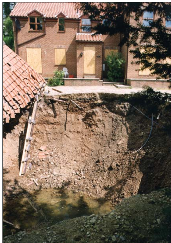
Figure 18 Solution collapse, affecting properties at Ripon Photo A. H. Cooper © NERC
