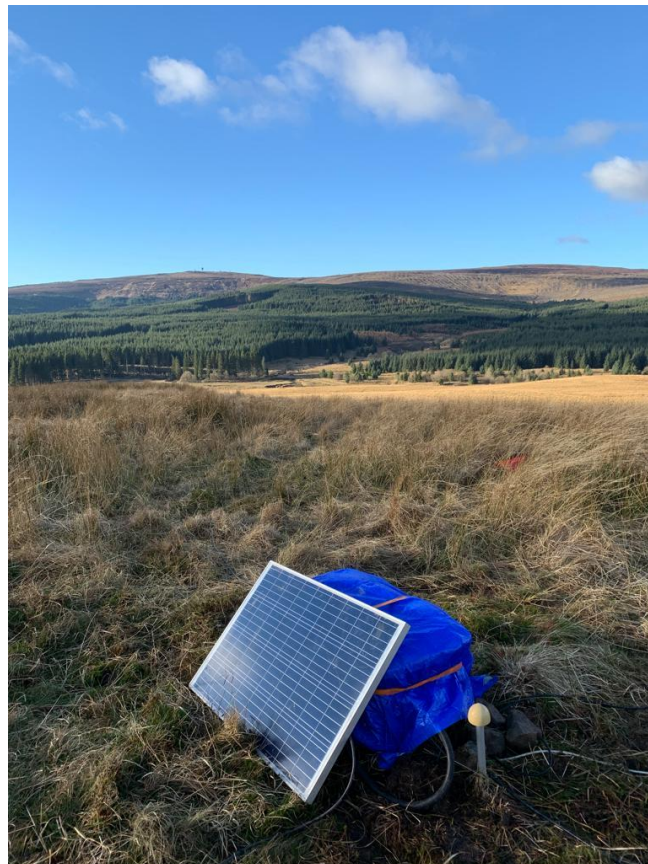
Figure 5: MT installation NY69 in Kielder Forest, Northumbria. All cables are buried to avoid interference from livestock. A small solar panel is constantly recharging the batteries. Visible is also the GPS antenna (white mushroom on a pole).
