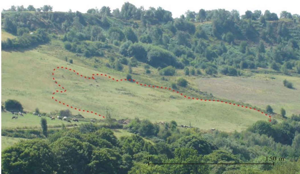
Figure 5: Shallow earth slide failure at SK290867. This failure occurs next to a more degraded, larger slide that is obscured by the trees. (Photograph taken from 429600 387831).
