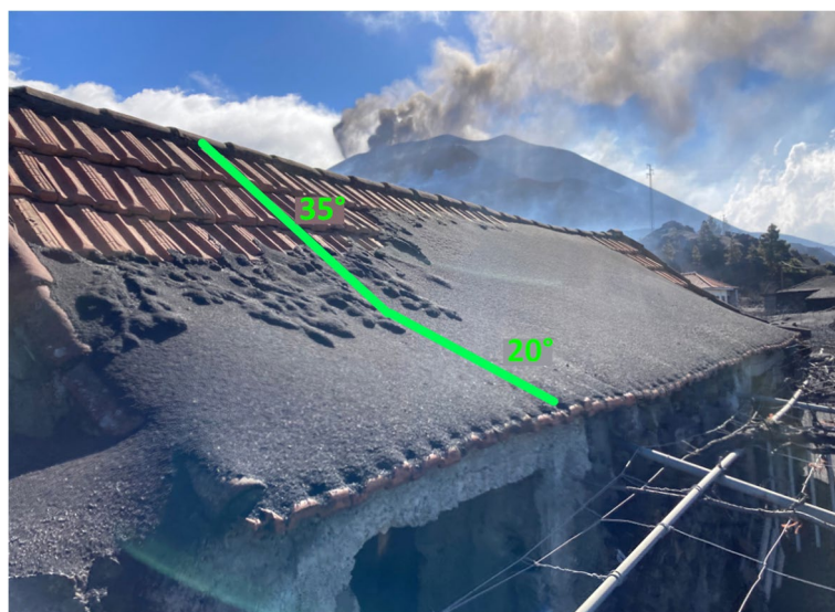
Fig. 11 Tephra deposit on a roof in Tacande, La Palma, December 2021 during the Cumbre Vieja eruption. Tephra has slid on the steeper part of the roof ( \sim 35^\circ pitch) but accumulated on the lower, shallower part ( \sim 20^\circ )
