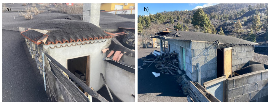
Fig. 9 Low pitched roofs in (a) Las Manchas and (b) Tacande, La Palma following the Cumbre Vieja 2021 eruption, showing no evidence of the deposit sliding except at the deposit edges where the angle of repose has been formed
