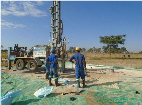
Drilling site in Zimbabwe
