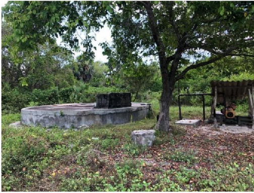
(a) Piped water supply scheme source
