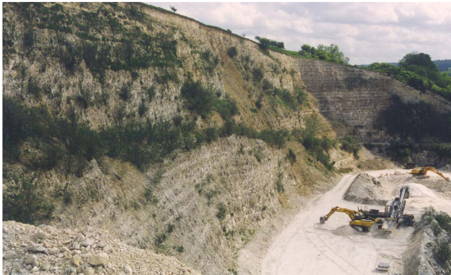
Plate 4. Somborne Lime Quarry. Chalk from the White Chalk Group is extracted for agricultural lime and low-grade aggregate. (GS 1098, P.M. Hopson)
