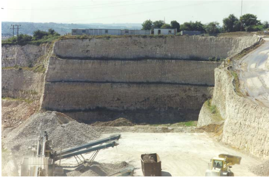
Plate 3. Warren Farm. A small quantity of chalk is extracted from the White Chalk Subgroup at Portsdown Hill. The pit is also used for recycling and waste disposal. (GS 334, P.M. Hopson)
