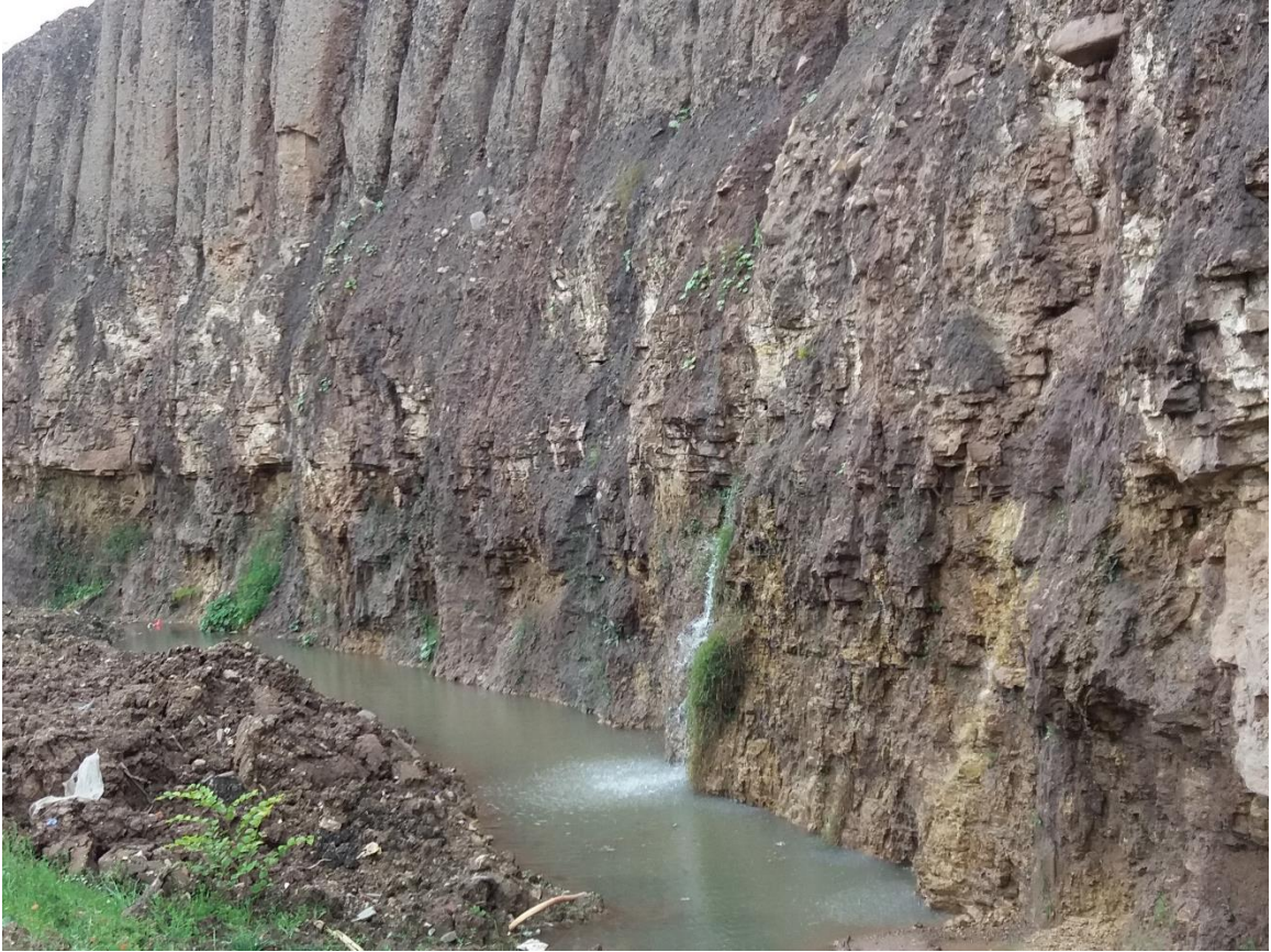
Figure 2 Springs at Aycliffe Quarry [NZ29524 22571].
