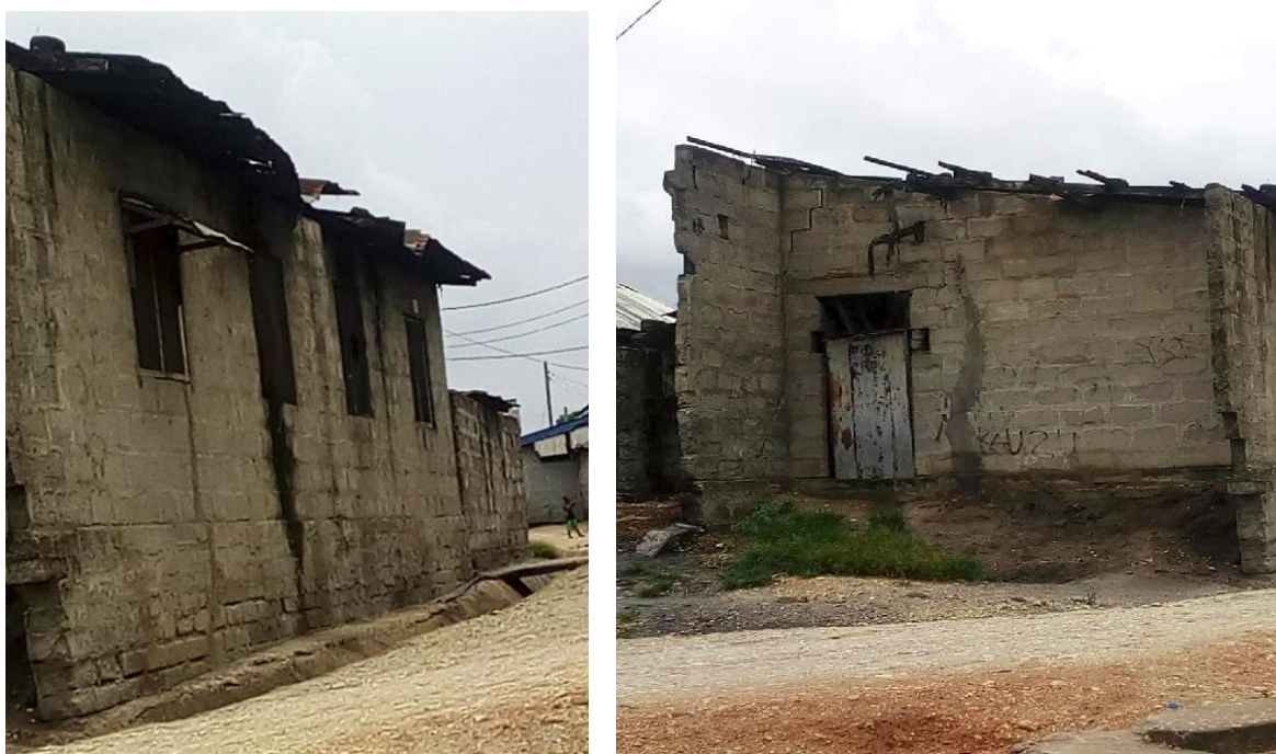
Figure 13: Building Photos © HOT Tanzania
