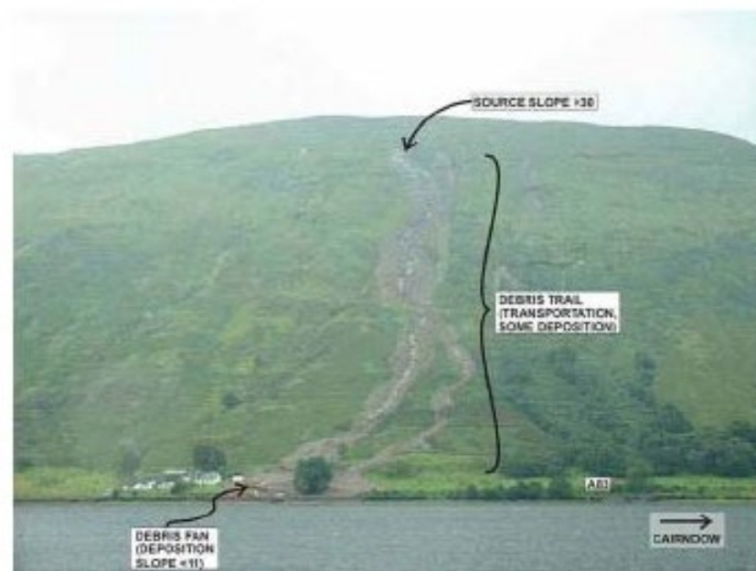
Main Characteristics of a debris flow on A83 Cairndow
