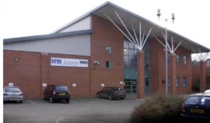
Underground sinkhole discovered under Ripon's new swimming pool
