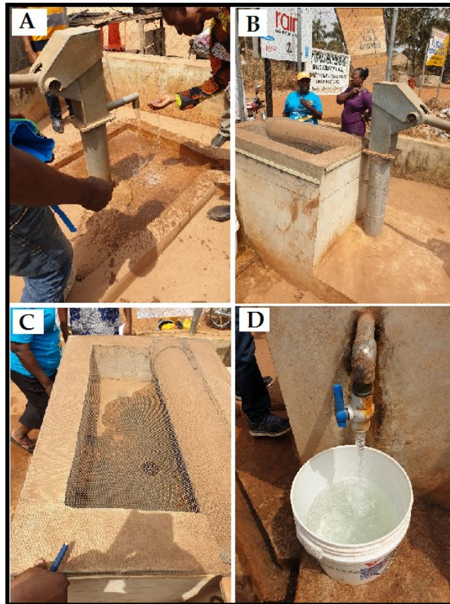
Figure 2. (A) One of the hand-pump wells without Iron filtration chamber at Ugwuaji community (B) One of the hand-pump wells with Iron filtration (C) Open Iron filtration/Ion exchange chamber at one of the wells. (D) Water collection point from one of the Hand-pumps.
