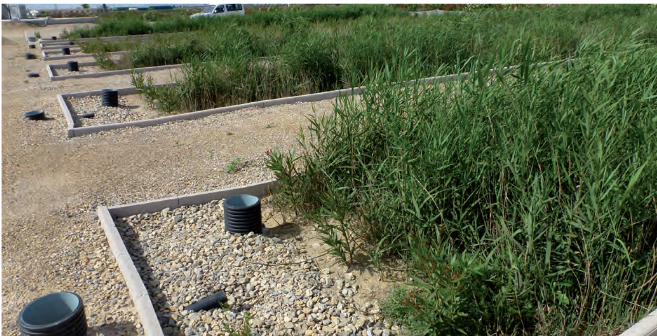
Image 29: Example of a constructed wetland for water treatment by nutrient removal using a paludal culture (common reed, Phragmites australis ) (Landscape Measure 6) (photograph: © Angel Faz, 2021).
