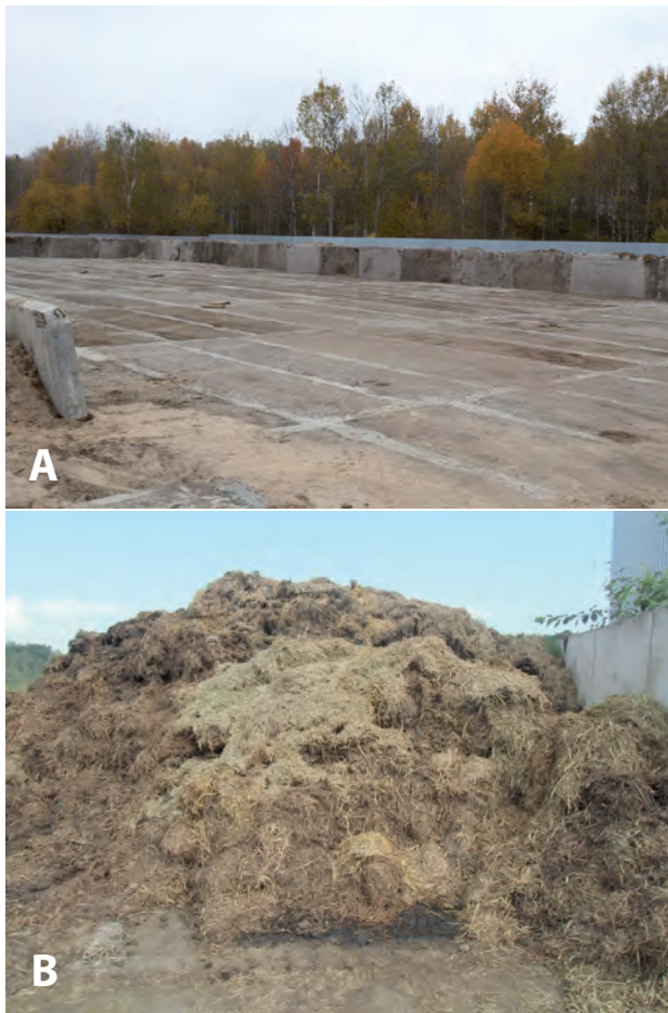
Image 11: Open storage of solid manure on a solid concrete base with walls (A, B; Manure Measure 5) helps reduce nitrate and other nitrogen leaching and run-off, but risks substantial ammonia emissions to the atmosphere (photographs: © Sergei Lukin).
