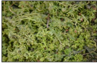
Disintegration and surface slime
