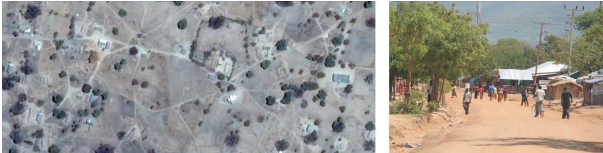
Figure 3.2: Development Pattern 1 in Tanzania. Left: GoogleEarth 1 , accessed in 2018. Right: available street level images.
