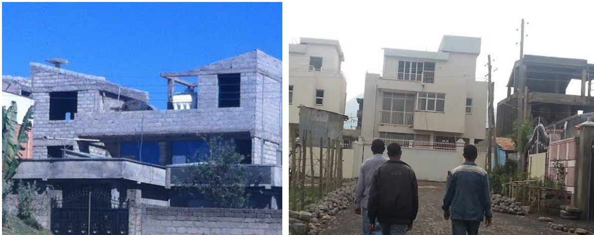
Figure 3.5: 3-story RC frame homes, from available street level images
