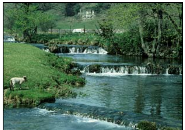
Figure 3. Wiers on the River Lathkill.
