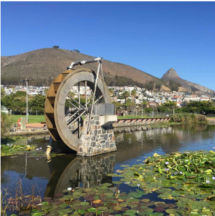
Reconstruction of groundwater fed municipal water infrastructure, now providing environmental and aesthetic benefits. Cape Town, South Africa.
