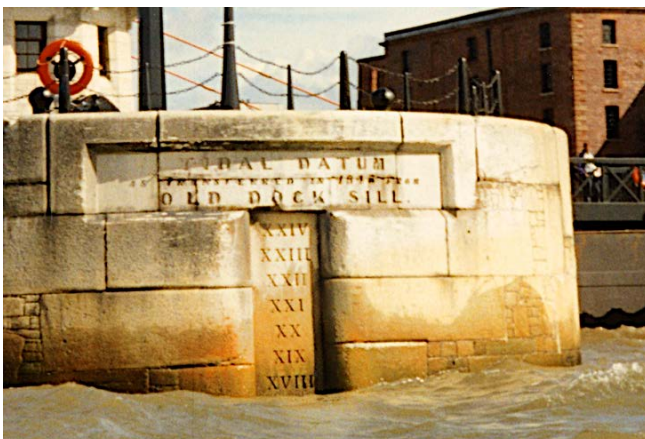
FIGURE 1. An example of a visual “tide gauge” engraved on a harbor wall, showing tide level markings at the entrance to Canning Half-Tide Dock, Liverpool, relative to the Old Dock Sill datum, a reference datum defined around 1715 in terms of the sill of Liverpool’s first dock. Photo credit: Philip Woodworth, National Oceanography Centre
