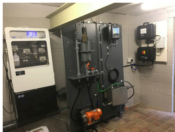
FIGURE 5.2 Automatic water quality monitoring station, Lower River Thames, UK. Photo credit: Mike Bowes.
