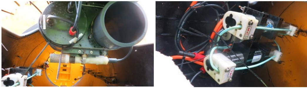
One of the CO 2 sensors and the microCATs on the DY116 buoy as recovered DY130
