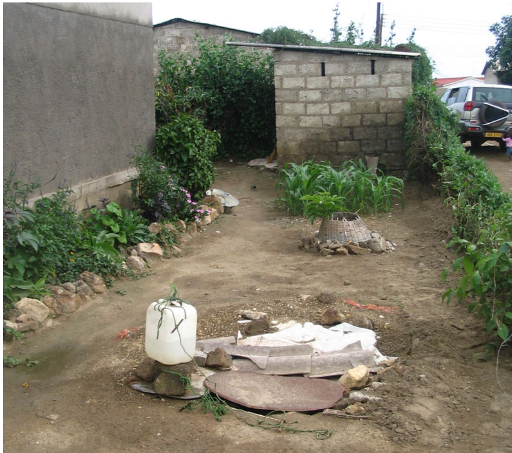
Fig. 6.12 Close proximity of groundwater well and pit latrine in peri-urban area of Lusaka, Zambia. Credit Kenedy Mayumbelo (reproduced under a CC BY 2.0 license)
